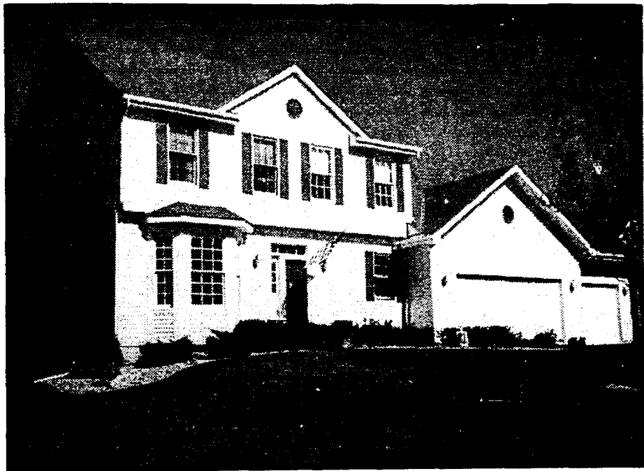
HEY GOOD LOOKIN'. New aluminum, vinyl, or steel siding gives existing homes an attractive exterior appearance, essential for wooing today's potential home buyers.
