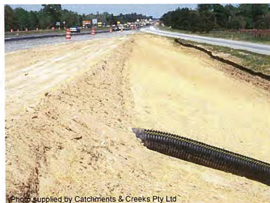
Photo 5 – Earth flow diversion bank used to direct runoff towards the entrance of a Slope Drain
