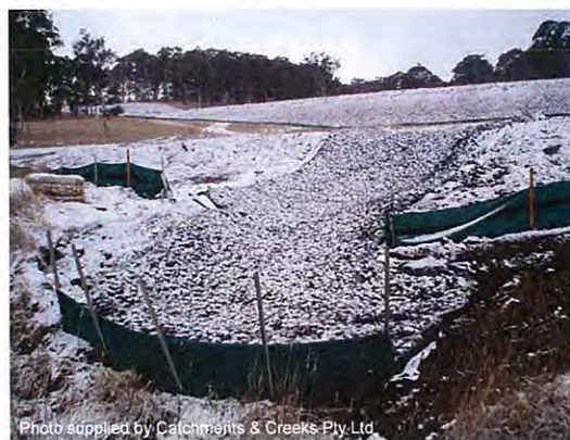
Photo 2 – Temporary rock mattress outlet structure at end of a Chute
