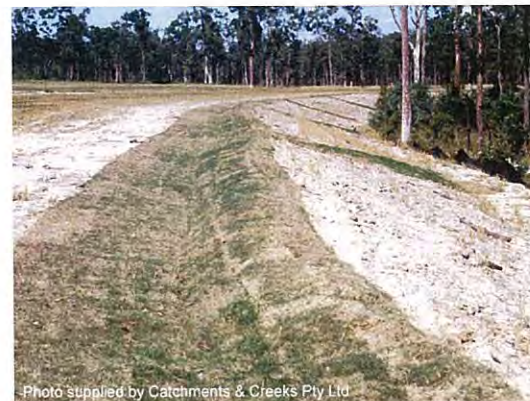
Photo 6 – Turf-lined flow diversion bank with grass-lined outlet chutes at regular intervals along the embankment
