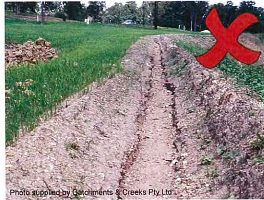
Photo 6 – Velocity-induced bed scour within a catch drain
