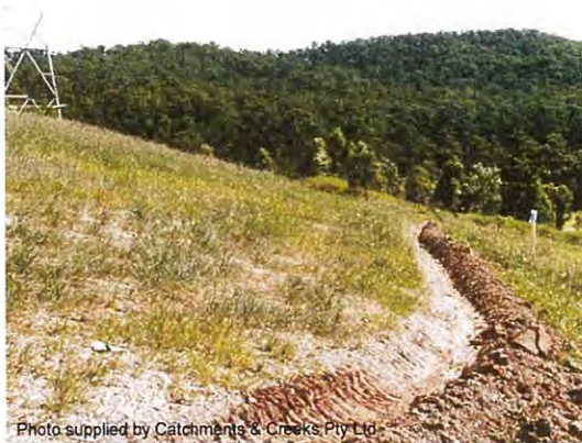
Photo 1 – Unlined catch drain
