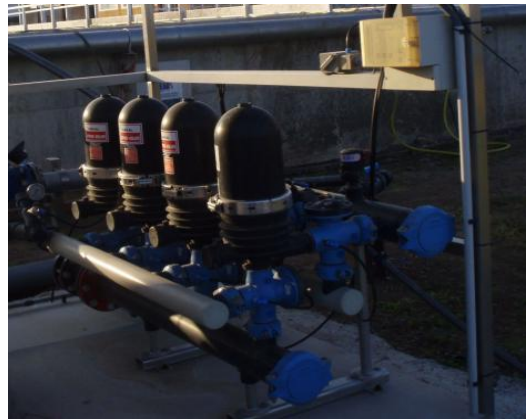
Figure 1. View of the ring filter.
