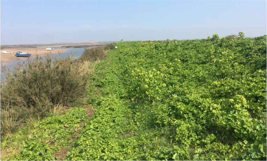
Fig. 1. Sea wall at Burnham Overy Staithe (P. Boardman).
