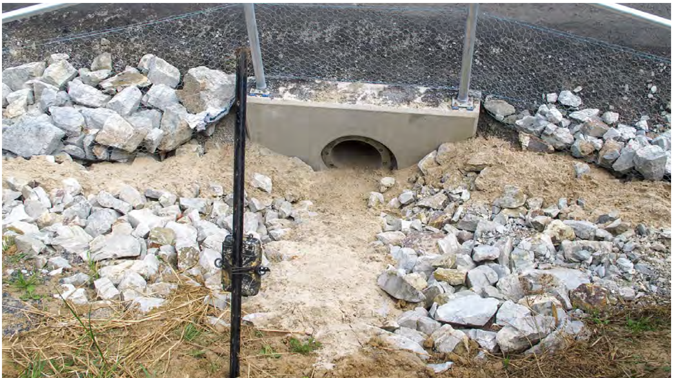
Figure 6: Photograph showing the sand and small gravel that was added to the culvert entrances as a transition from the riprap to the smooth concrete of the culverts. A camera trap is shown in situ. Photograph ©2018 Peter Vertigan
