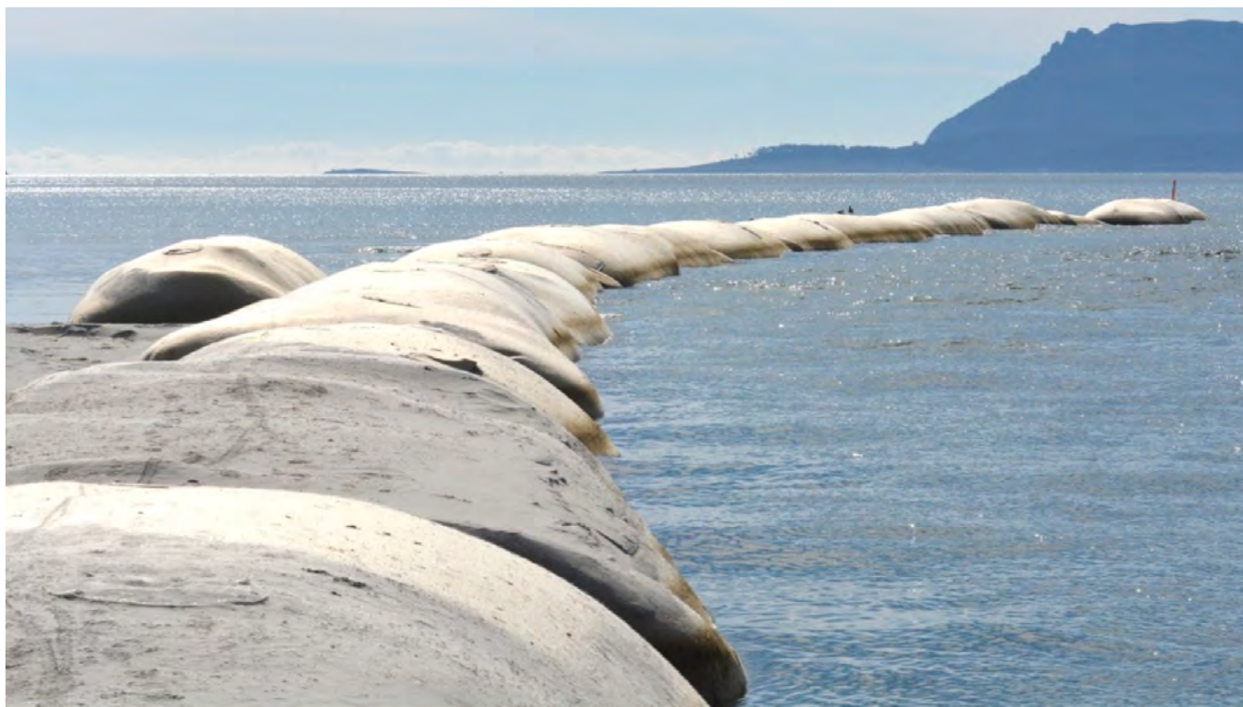
Figure 16: Bag placed adjacent to main channel alignment to seal a gap between bags (Maria Island in the background), 30 November 2017. ©Eric J. Woehler
