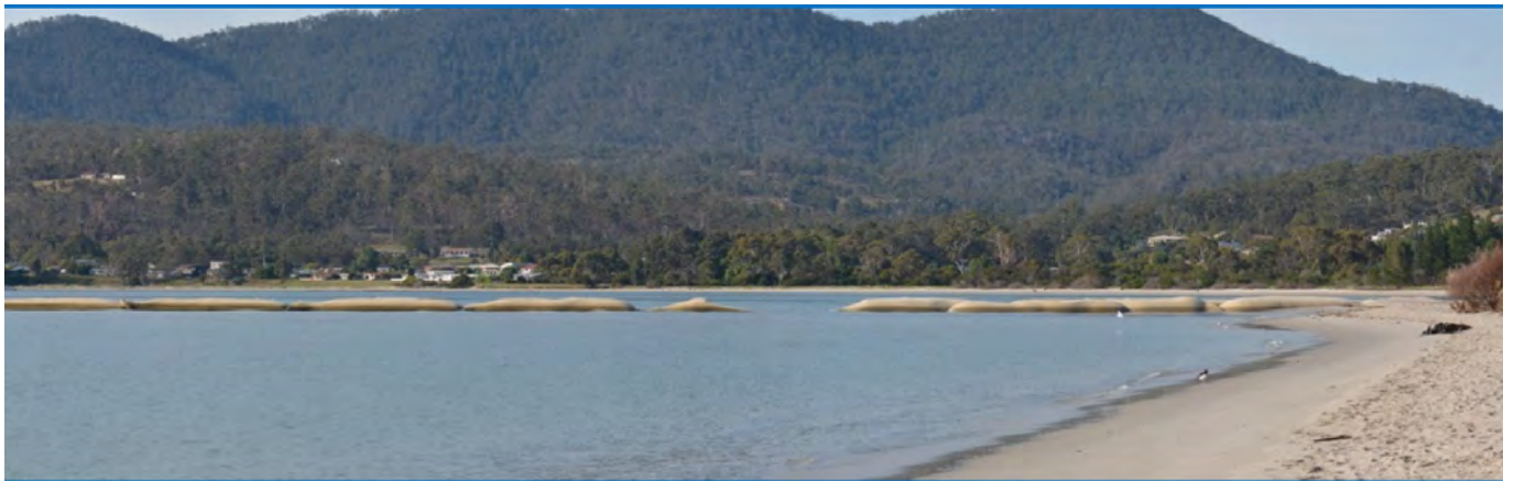
Figure 15: Gaps in the constructed channel at the mouth of the Prosser River, 30 November 2017. ©Eric J. Woehler
