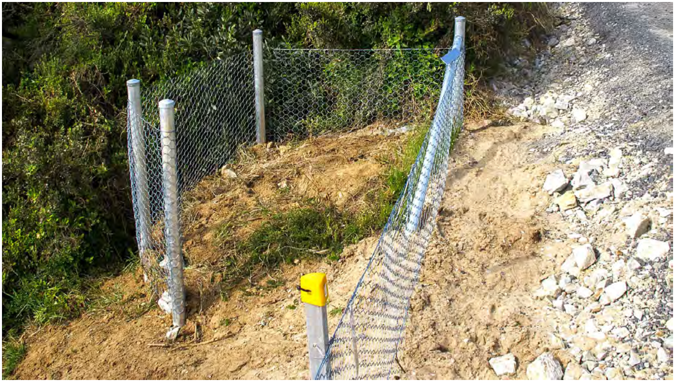
Figure 5: Photograph showing the square 'return' that was added to the ends of the fences to guide the penguins through 180° back towards the culvert entrances within the fencing extent. Photograph ©2018 Peter Vertigan
