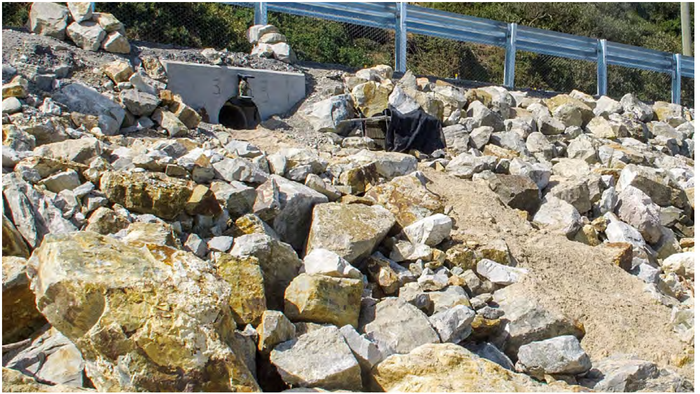
Figure 7: Photograph showing the path through the rearranged riprap material below the culvert entrances with beach sand placed to form a pathway to direct penguins towards the culvert entrances. Photograph ©2018 Peter Vertigan
