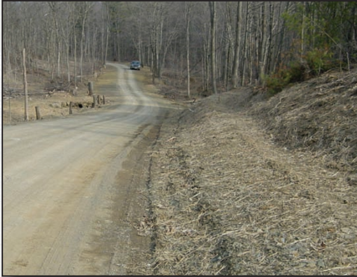
Figure 7.10—The slightly insloped bench in this image takes the water around the hill and away from the road.
