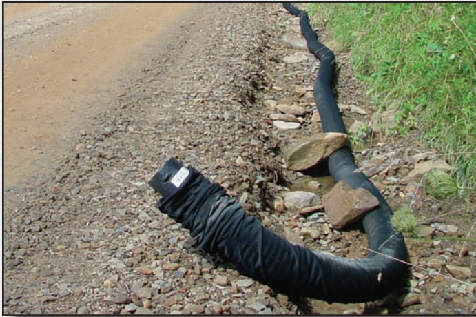
Figure 2.6—Perforated plastic pipe.
