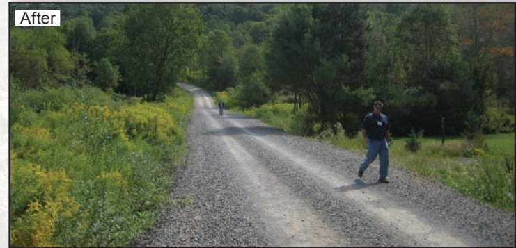
Figure 2.17 and 2.18—This roadway cuts across a flood plain wetland. A 300-foot-long French mattress was used to provide relief for wetland flows while providing a stable road base and preventing beavers from damming the nearby stream pipe.
