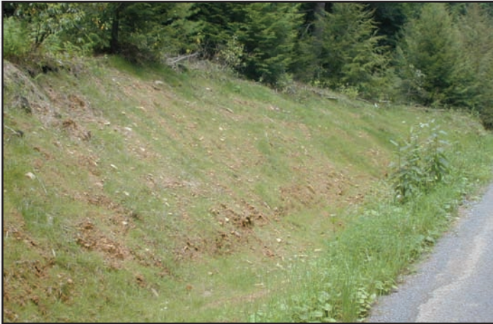
Figure 7.2—Trying to grow grass on a smooth bank made of subsoil and rock is not a good strategy.
