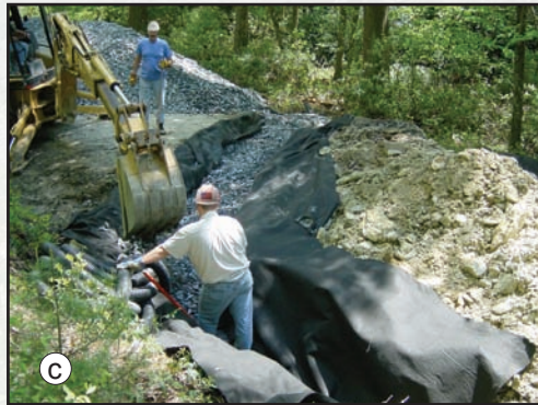
Figures 2.8a through 2.8d—French drain construction sequence.
