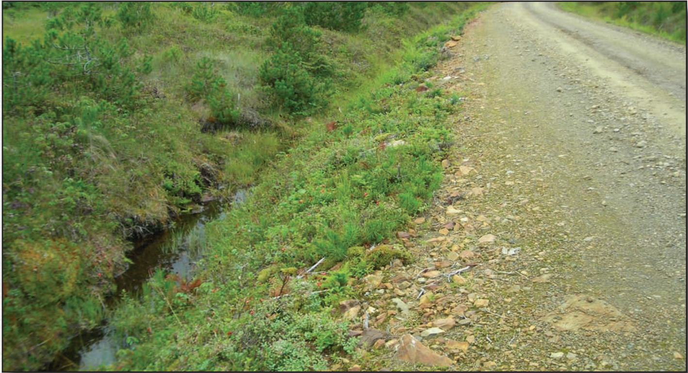
Figure 2.1—Permeable fill provides for subsurface flows.
