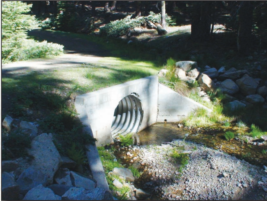
Figure 5.14—Headwall with wingwalls.
