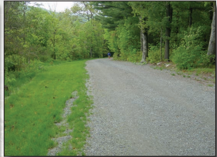
3.4b—Outsloped roads eliminates ditches.
