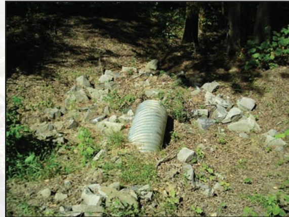
Figure 5.3—Culvert outlet is well armoured.
