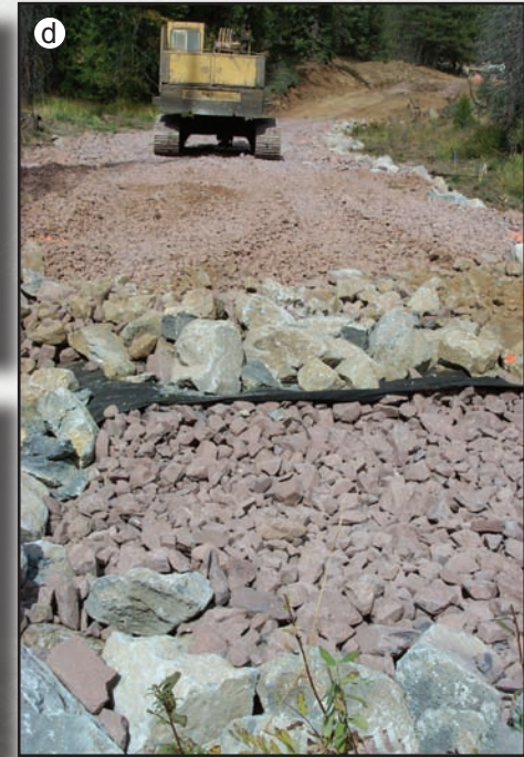
Figures 2.22a through 2.22d—Permeable fill construction sequence.
