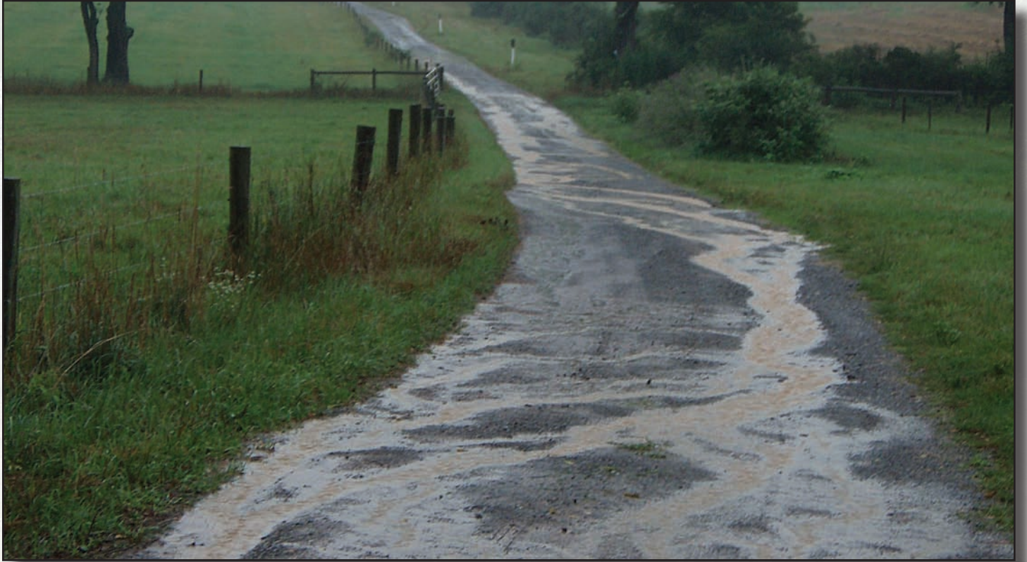
Figure 3.1—The road cross-section should be designed to shed water from the road surface.
