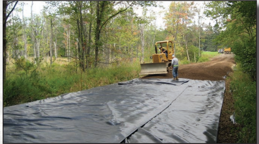
Figure 2.23—Geotextile fabric provides support for permeable fill.
