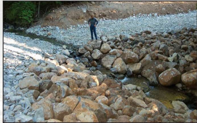
Figure 6.9—Boulder ford on Stanislaus National Forest in California has had no maintenance since construction in 1997.
