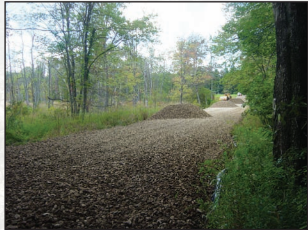
Figure 2.15b—Large mattress allows wetland flow.
