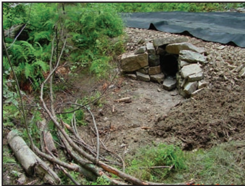
Figure 5.6—Shallow pipe. Placing the outlet at the natural ground elevation reduces maintenance and helps disperse flows.
