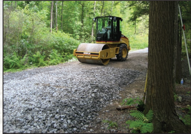
Figure 2.25—Roller compacts each of lift aggregate.
