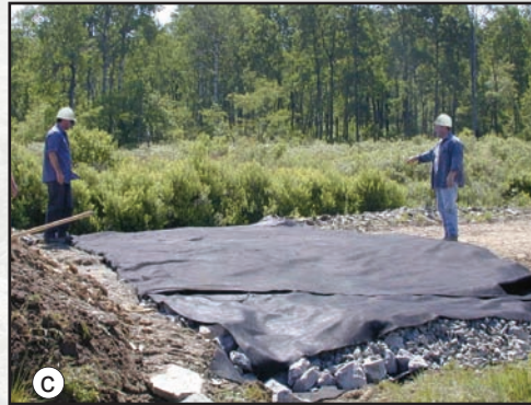
Figures 2.16a through 2.16d—French mattress construction sequence.
