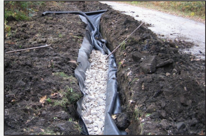
Figure 2.7—Free draining stone.
