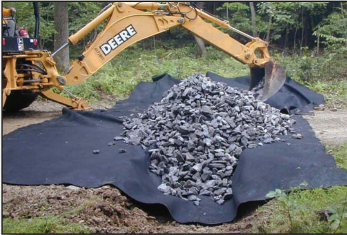
Figure 2.13—This small mattress was built to accommodate several springs and seeps that saturate the road each spring.
