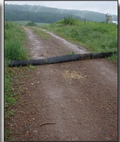
Figure 3.13—Conveyor-belt diversion on a farm lane (road).
