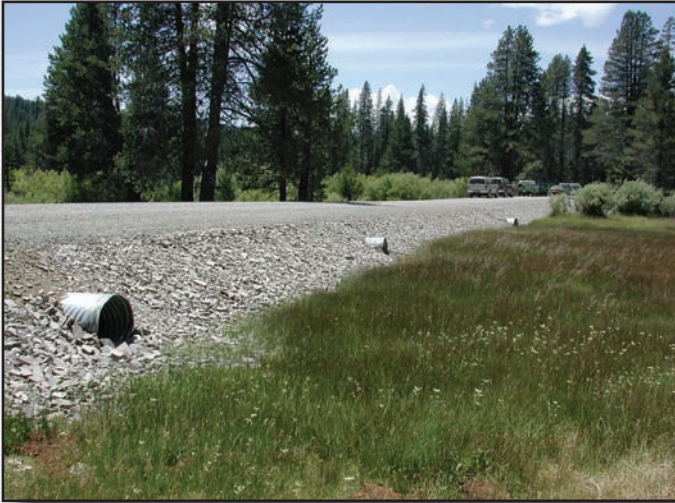
Figure 2.20—Permeable fill with culverts.
