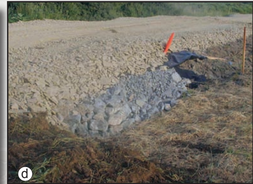
Figures 2.16a through 2.16d—French mattress construction sequence.
