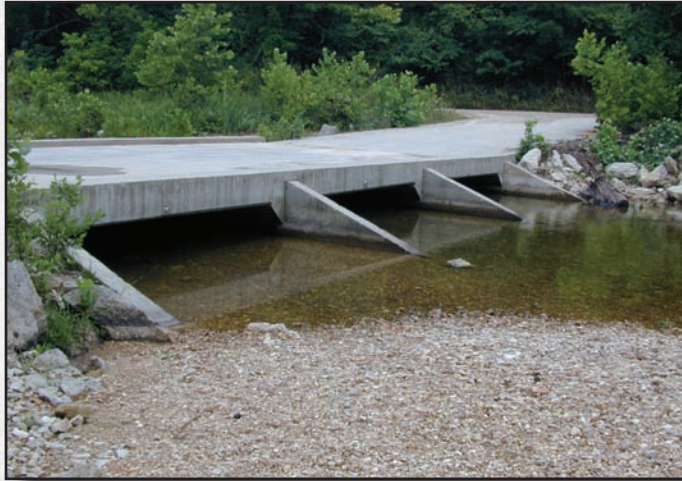
Figure 6.7—Vented ford or low-water bridge.
