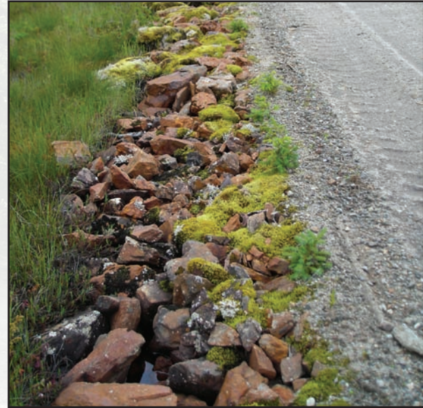
Figure 2.21—Permeable fill without culverts.
