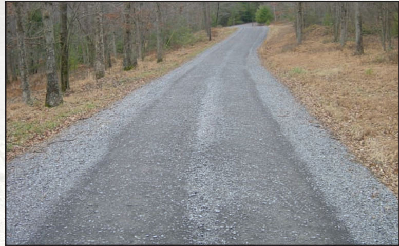
Figure 8.4—Loose aggregate will unravel and form windrows of material along the road center and edge.
