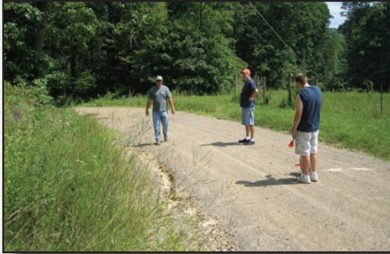
Figure 4.5—Near the top of a hill, this ditch is starting to erode. The team looks for drainage options.
