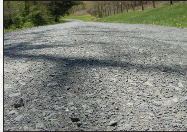
Figure 8.3—3-year-old dense packed surface aggregate after 40,000 vehicles.
