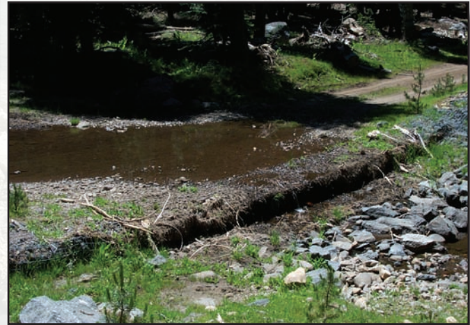
Figure 6.8—Gabion ford crossing.
