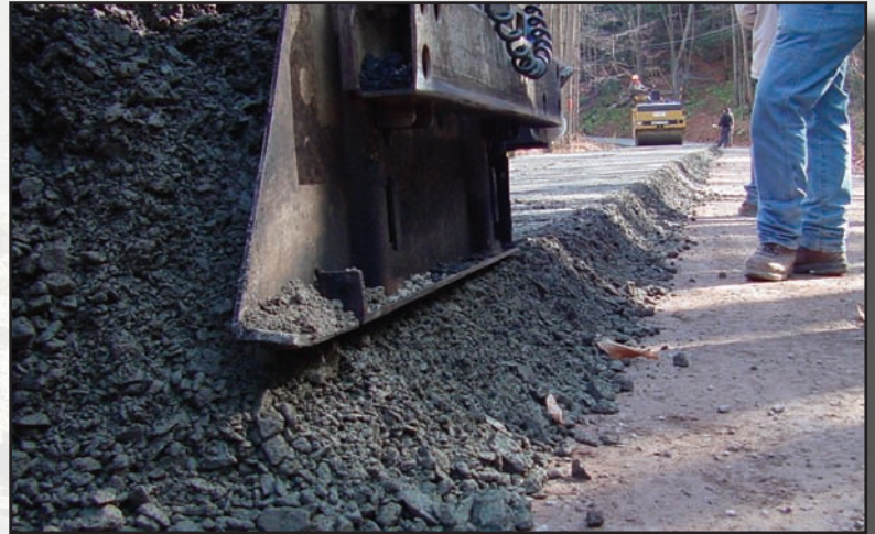
Figure 8.5—A well-graded aggregate is being placed through a paver at a noncompacted depth of 8 inches, and compacted to 6 inches. Notice the roller in the background for compaction.
