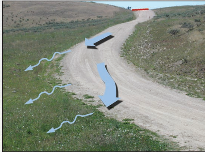
Figure 3.4a—Outsloped road disperses flow.
