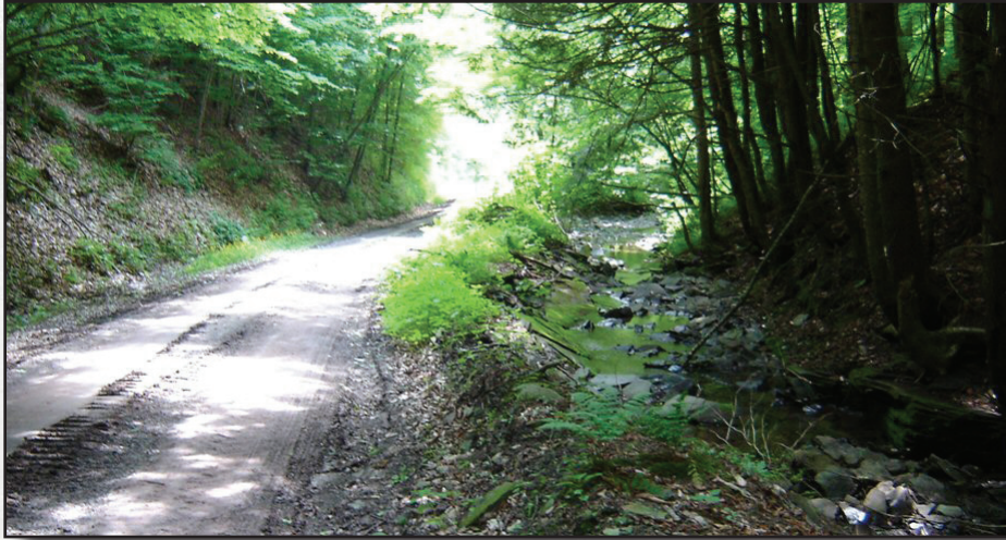
Figure 6.14—This road is constantly being eroded and flooded. Relocating the road away from the stream, while initially costly, will pay for itself in a few years of reduced flooding and repair costs.
