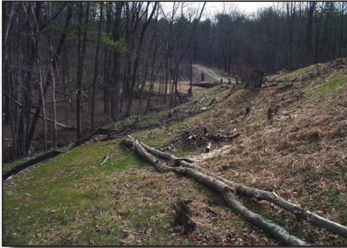
Figure 7.4—All of the woody debris and stumps in this picture were placed there to naturalize the bank shape.
