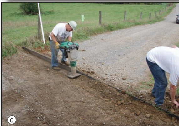
Figures 3.18a through 3.18d—Belt diversion construction sequence.
