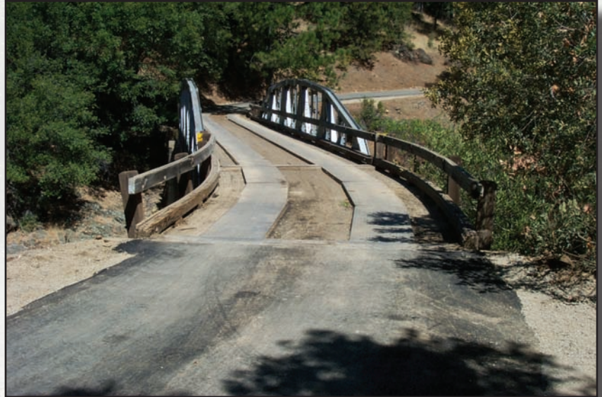
Figure 6.13—Paved bridge approach reduces sediment delivery to the stream.
