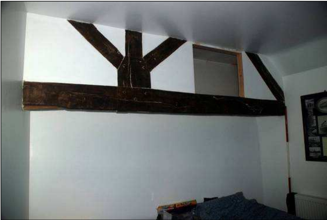
Plate 28: Truss 7 looking north
