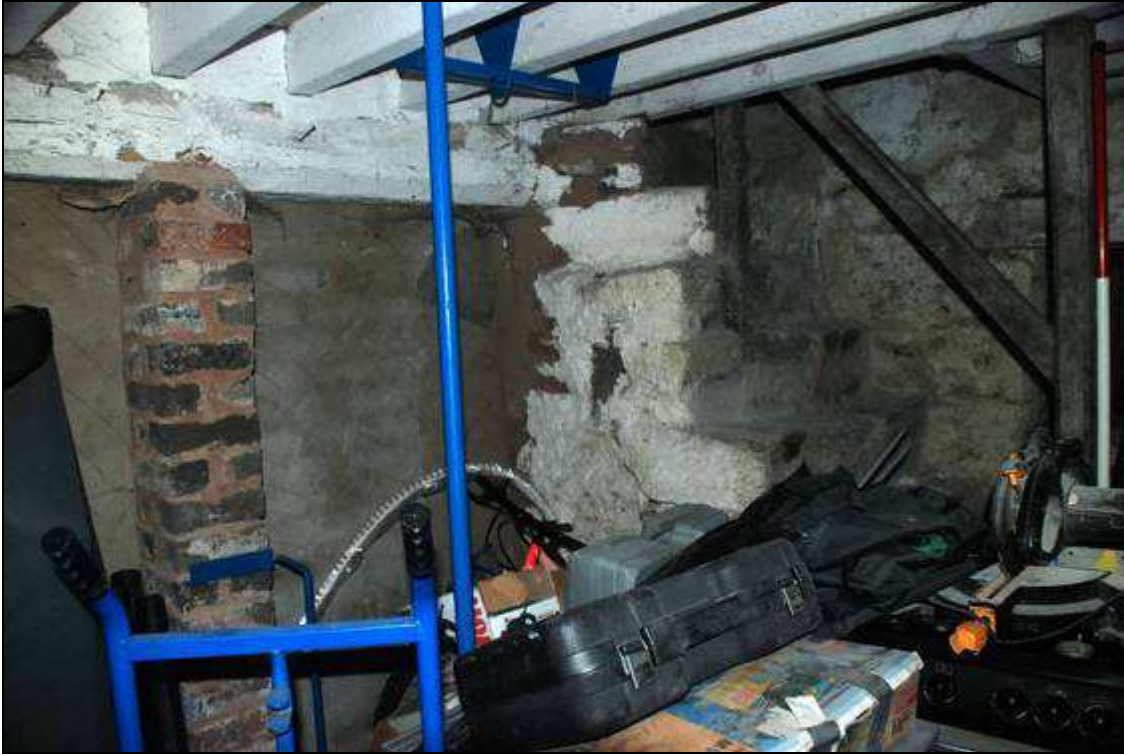
Plate 27: Staircase in the SW Wing, looking south
