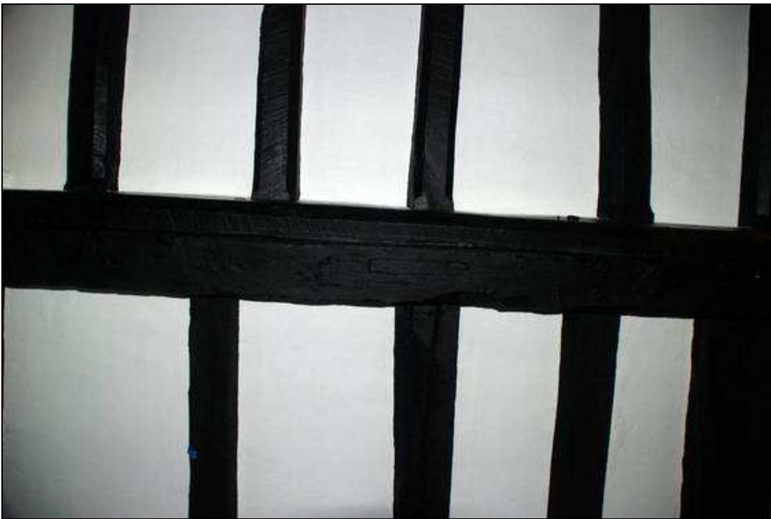
Plate 36: Underside of ceiling beam in NW room of main range
