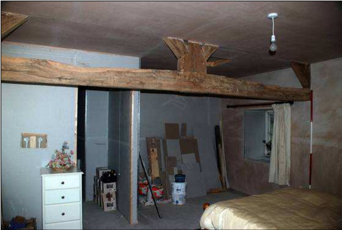
Plate 29: Base of Truss 8, looking north
