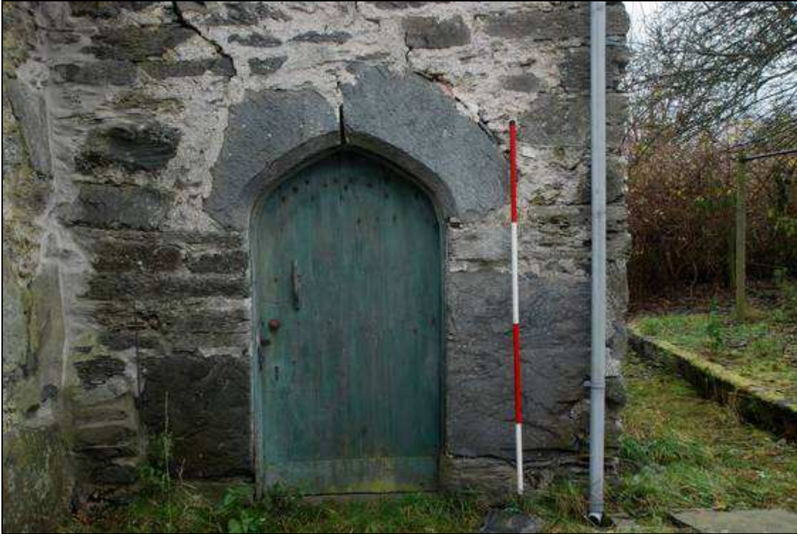
Plate 13: Door to the SW wing, looking SW
