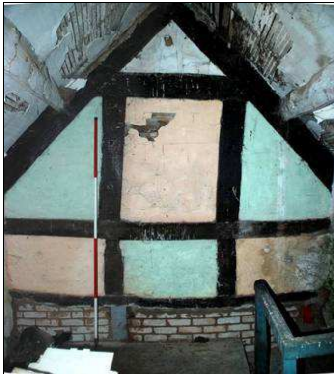
Plate 26: Partition between the main range and SW Wing, looking SE
