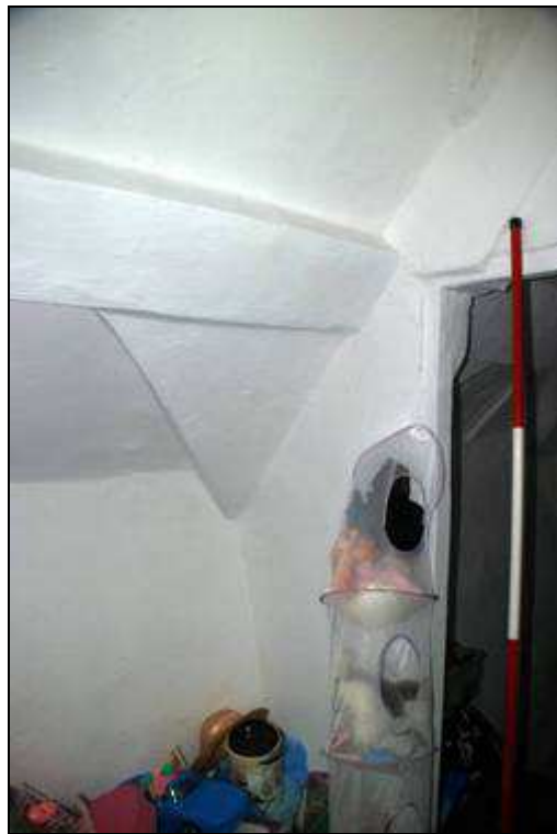
Plate 20: Windbrace between the lower purlin and Truss 2, looking north
