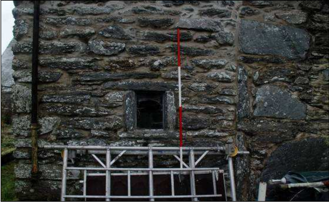
Plate 11: Small window in the SW range, looking NE
