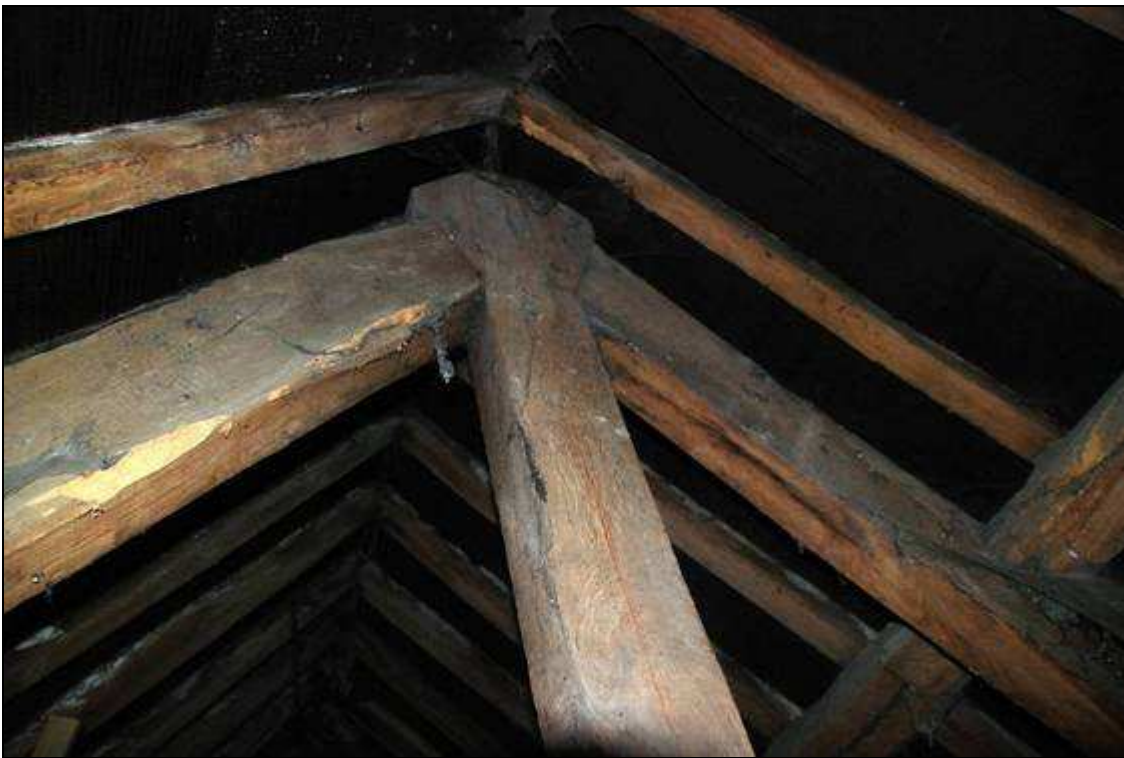
Plate 30: Top of Truss 8, looking SE
