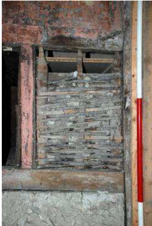
Plate 50: Woven lath panel in partition over stairwell, looking SW
