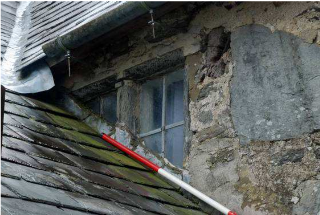
Plate 6: Window partly blocked by later extension, looking east
