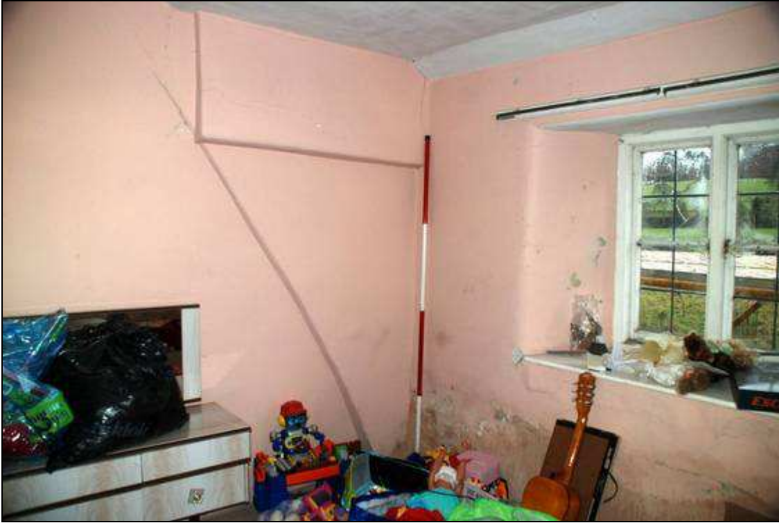
Plate 19: Truss 1, looking east
