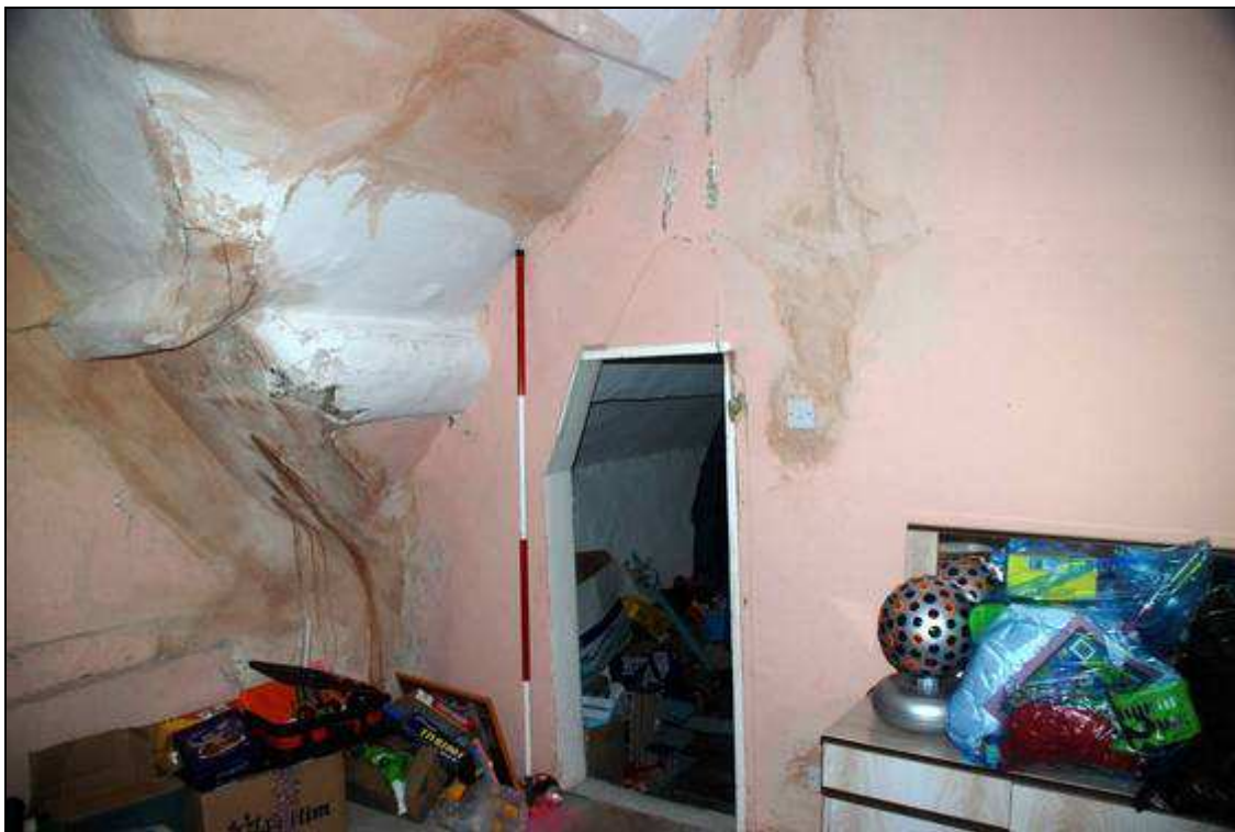
Plate 18: Truss 1, looking north
