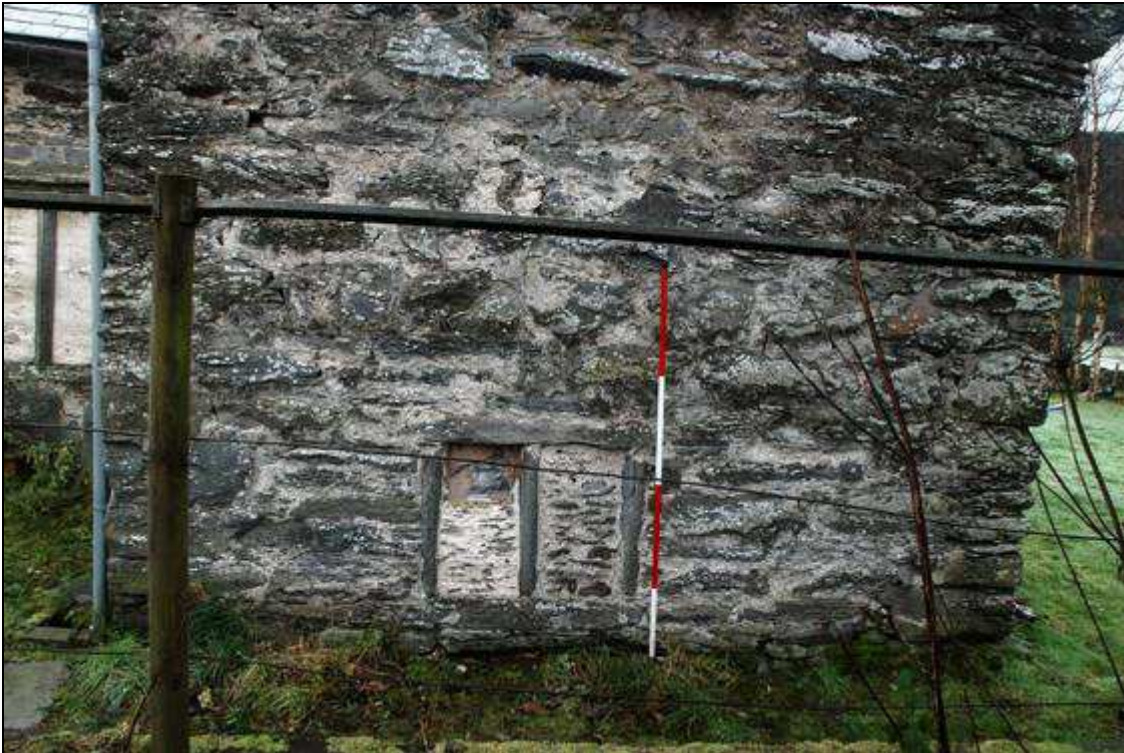
Plate 12: Mullioned window in SW range, looking SE
