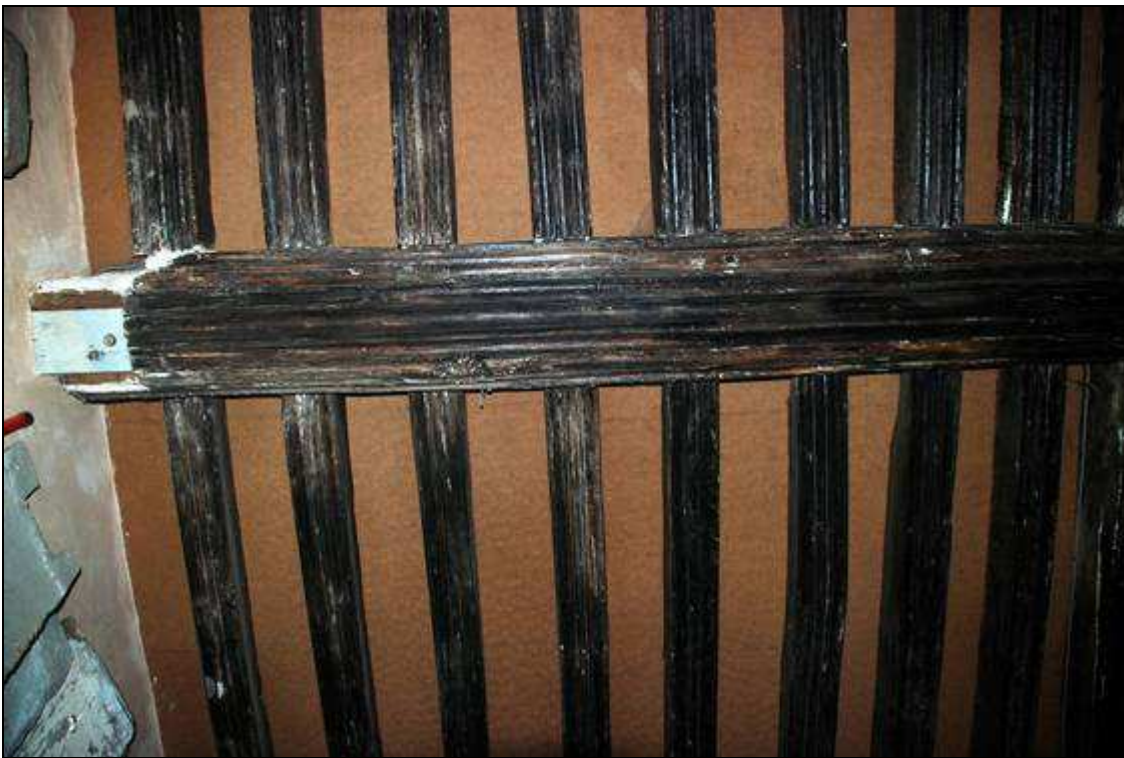
Plate 42: Moulded beam and joists in SW ground floor room, looking up
