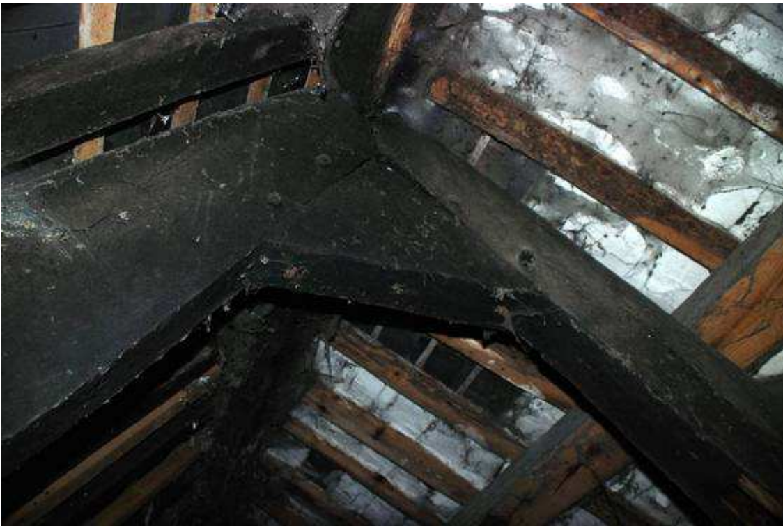
Plate 24: Straight insert at the peak of Truss 3, looking SW
