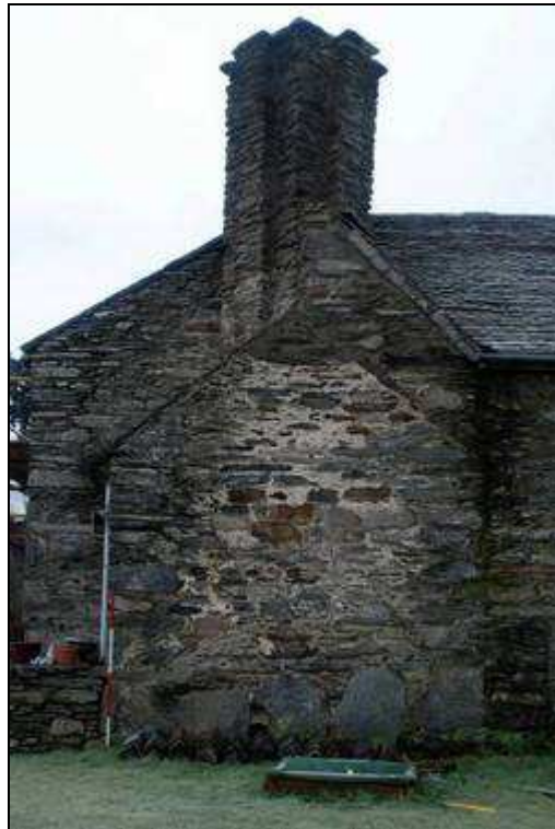
Plate 2: North eastern gable end chimney, looking SW
