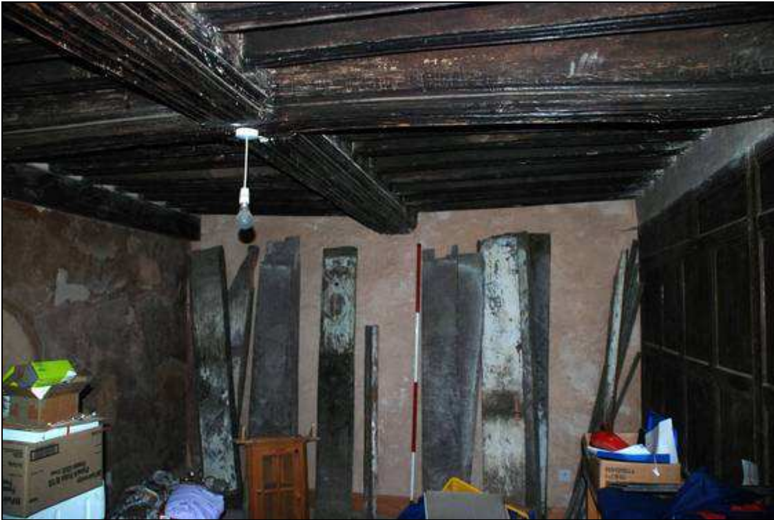
Plate 41: SW ground floor room, looking NW
