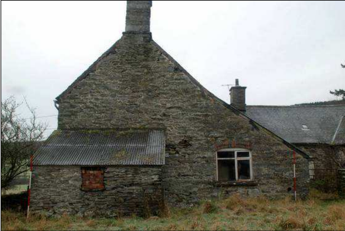
Plate 15: NE wing, looking SE
