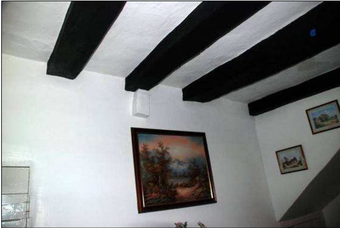
Plate 37: Sawn off joist in NE ground floor room, looking west
