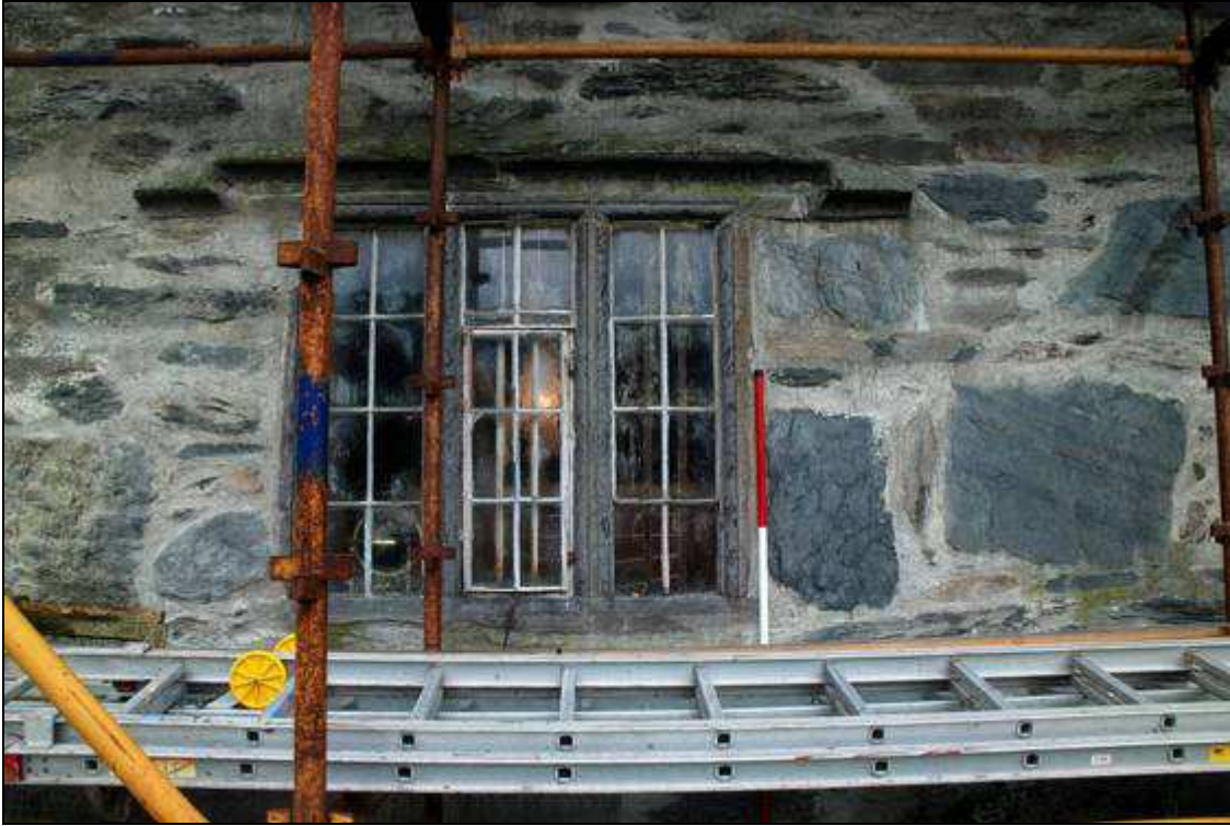
Plate 3: Three light mullioned window, looking NW
