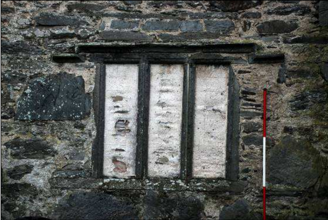
Plate 5: Blocked window, looking SE
