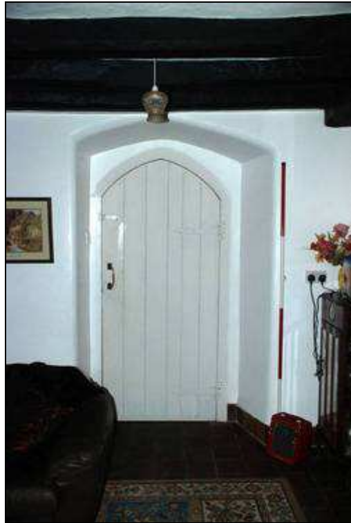
Plate 9: Door between main range and the kitchen, looking NW
