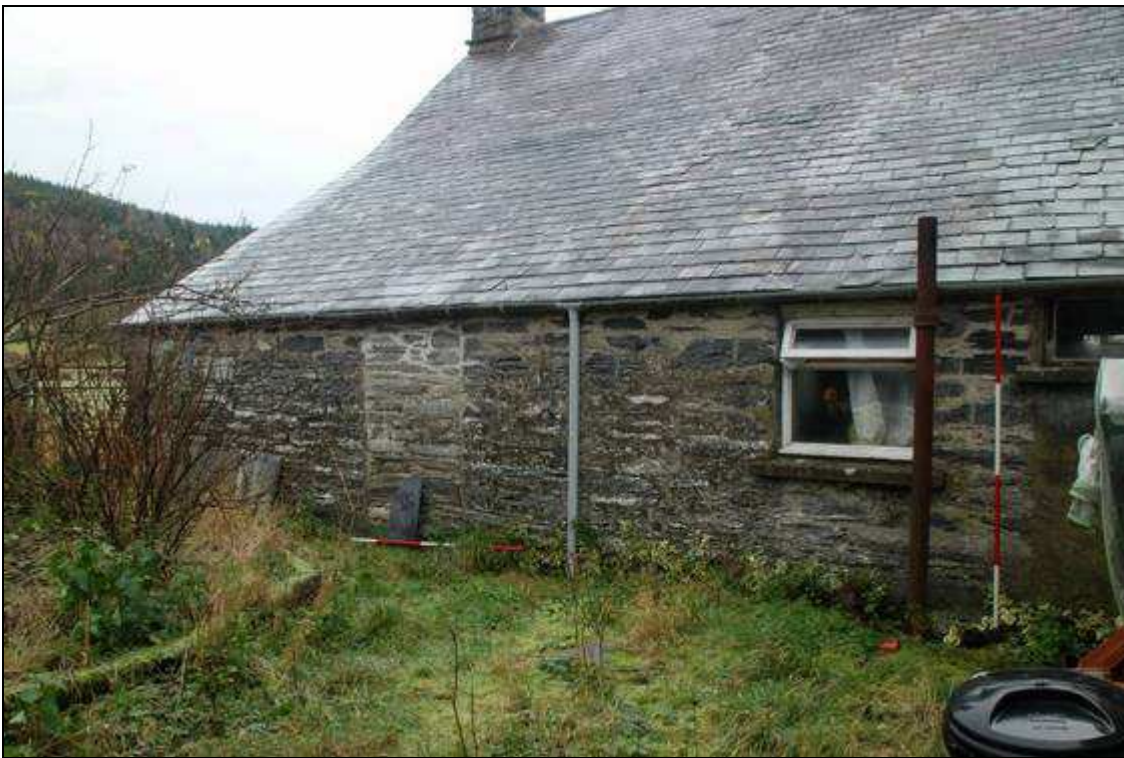
Plate 16: NE wing, looking NNE
