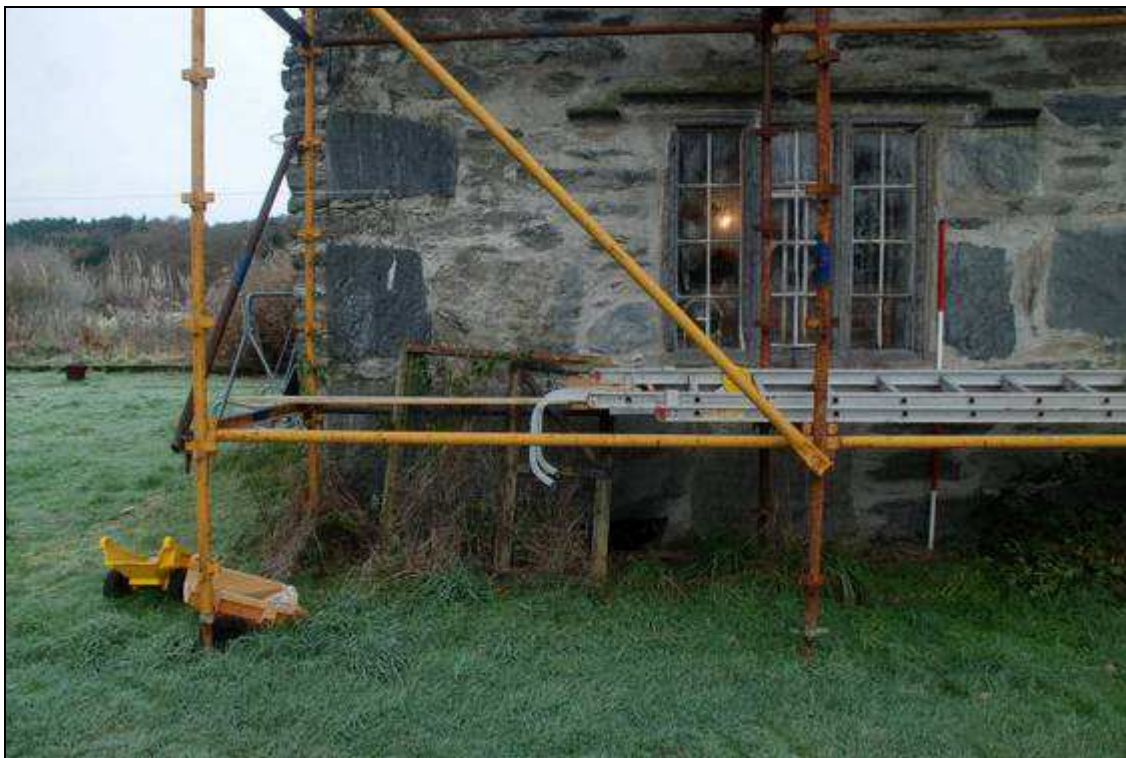
Plate 10: Cellar light and three light mullioned window, looking NW
