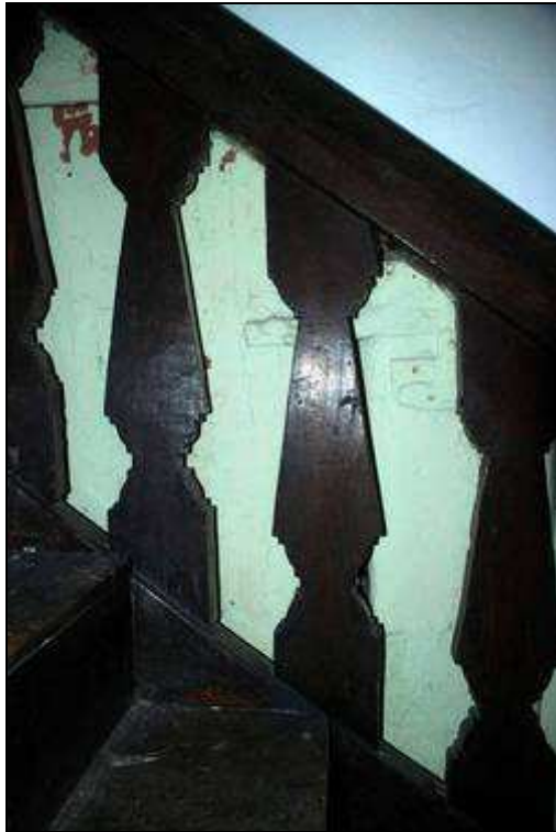
Plate 33: The splat balusters, looking SE
