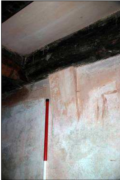
Plate 39: Foot of Truss 2, looking SE
