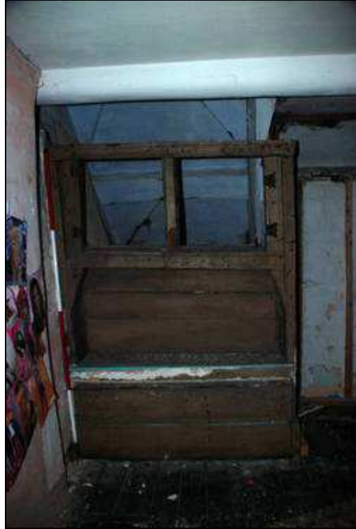
Plate 49: Partitioned shelf over the stairwell, looking NW
