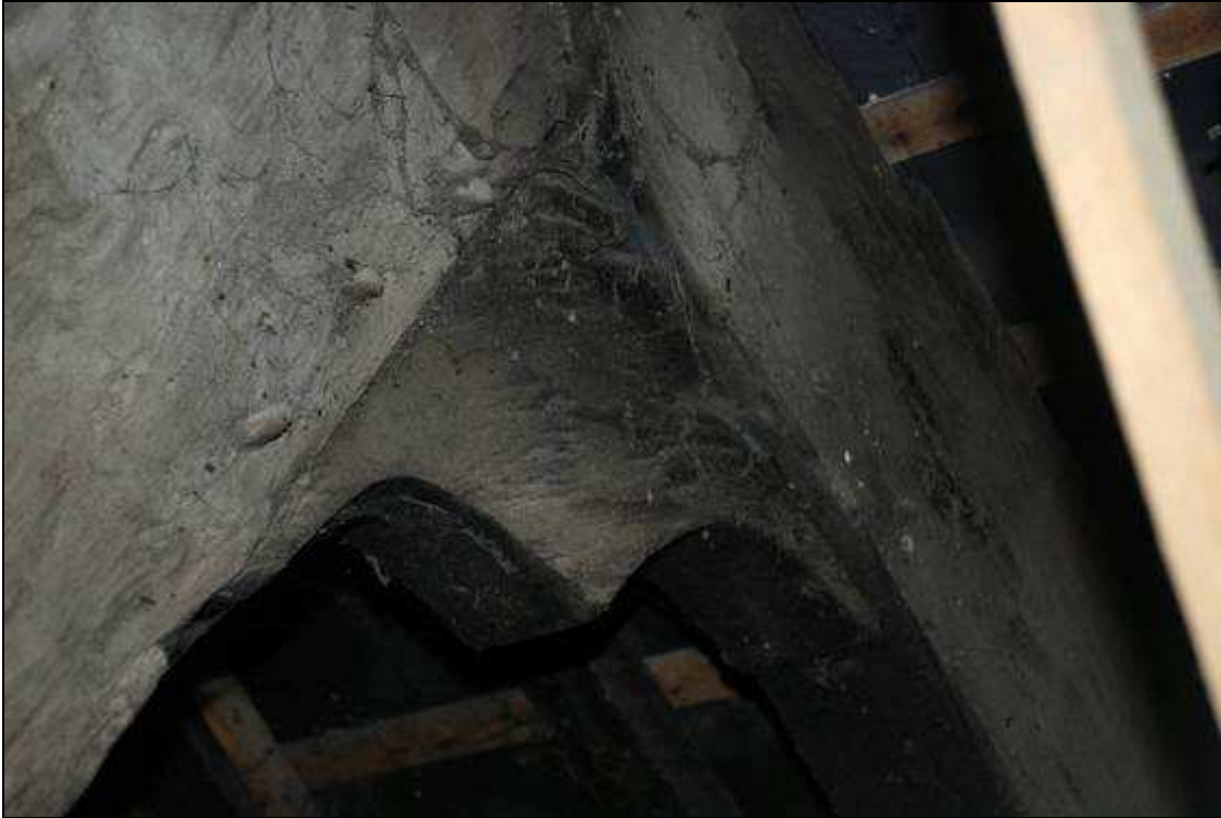
Plate 23: Cusped insert at the peak of Truss 2, looking west
