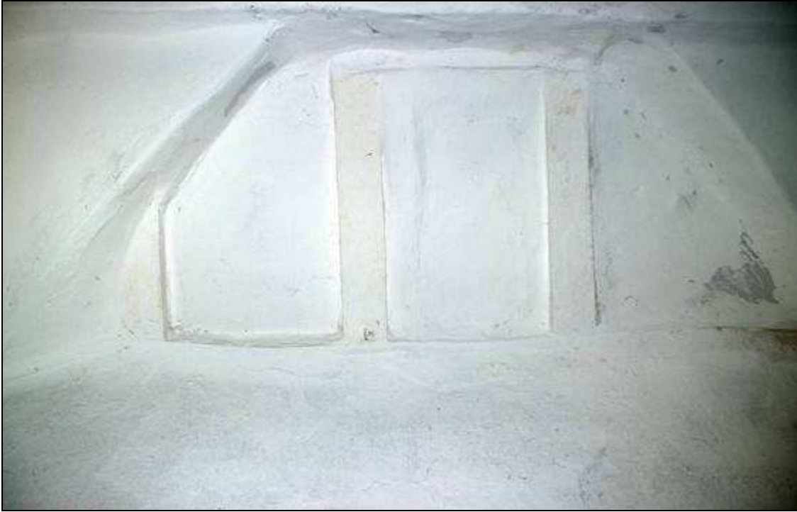
Plate 21: Windbraces and common rafters between Trusses 2 and 3, looking NW
