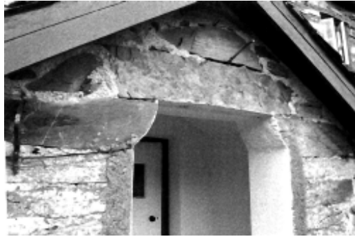
The front door – slate stone lintel on quarter round corbels
