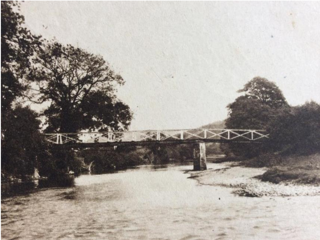
Pont Gwerclas between Gwerclas and Hafod y calch – now sadly washed away!
