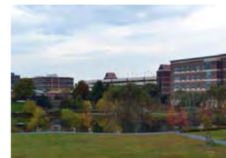
Valley Health Hospital 100+ MOBOTIX Kameras, USA
