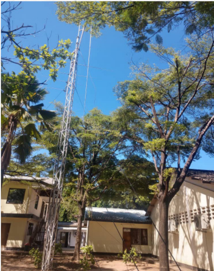
Radio Transmission tower at DIT done by the Company
