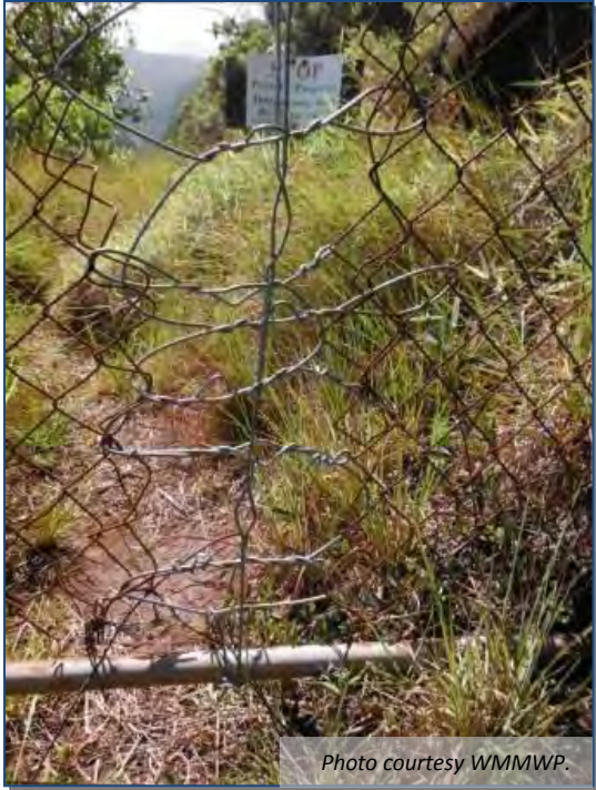
Figure 11. The Honokōwai ditch gate was vandalized in FY12, and repaired with fencing material.
