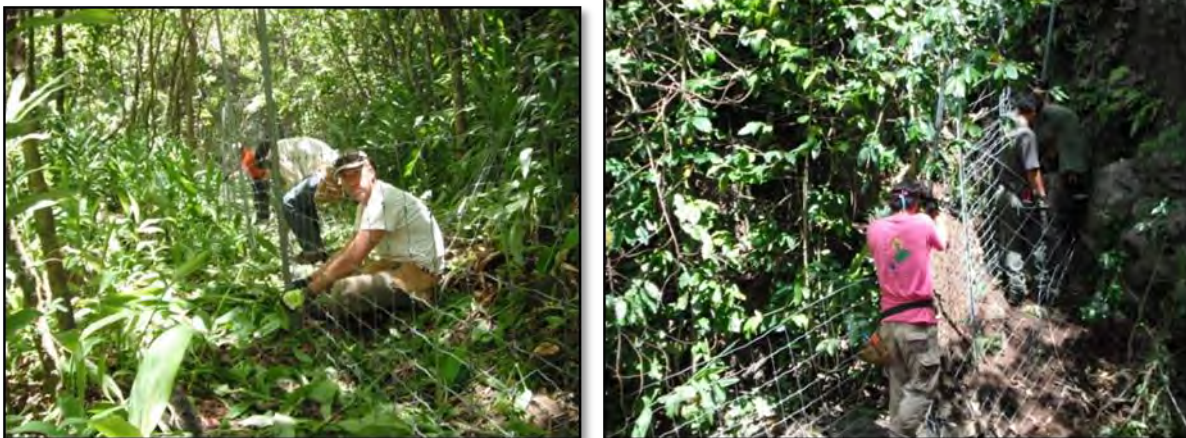
Figure 6. New Honokōwai Valley fence installed in FY14.
