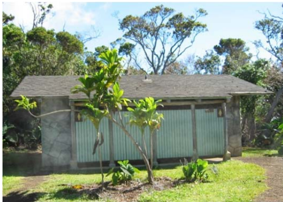
Photo 7-9 Kalalau Lookout Restroom
