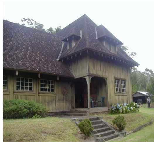
Photo 4-5 Danford House (TMK: 1-4-03: 13)
