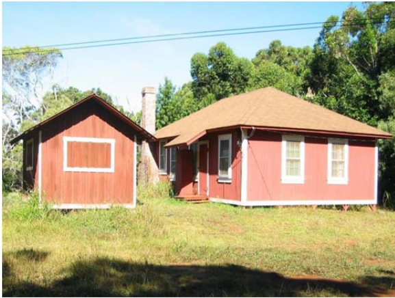
Photo 4-4 Hip Roof and Double-Hung Windows Līhu‘e Plantation Company Cabin (TMK: 1-4-02: 48)
