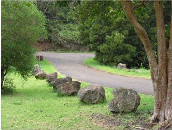
Photo 7-18 Boulder Bollards Detail Kōke'e Campground, Kanaloahuluhulu
