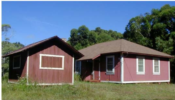
Photo 7-2 Typical Roof Architecture – Gable (right) and Hip (left), Composite Material TMK: 1-4-02: 48
