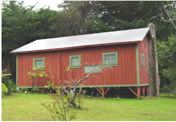
Photo 7-1 Kōke‘e Vernacular: Board and Batten, Post-on-Pier Foundation, Corrugated Gable Roof, Wood-framed Glass Pane Windows TMK: 1-4-04: 09
