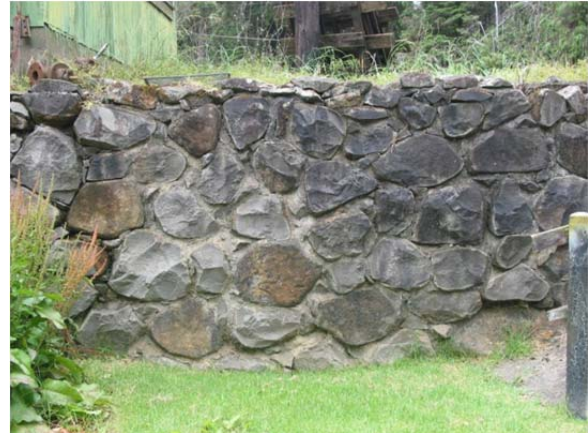
Photo 7-6 Stone Wall Detail CCC Camp Base Yard
