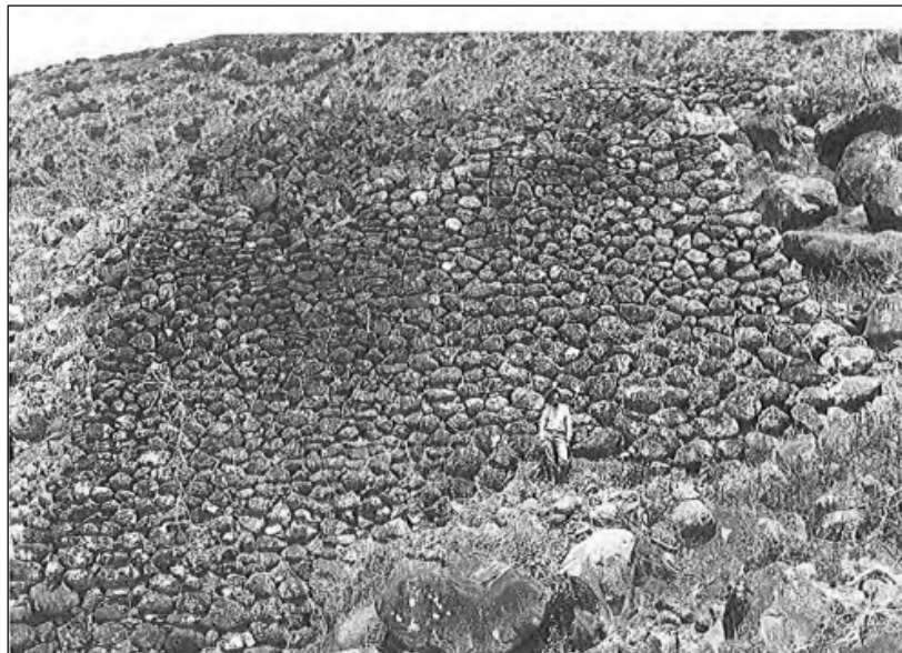
Figure 34. Eastern retaining wall of Kaluakapi'ioho Heiau (Site 175). The wall is 11 m (36 ft.) high at the southern corner and 8 m (26 ft.) high on the northern corner. Photo by Stokes (1909) as illustrated in Summers (1971).
