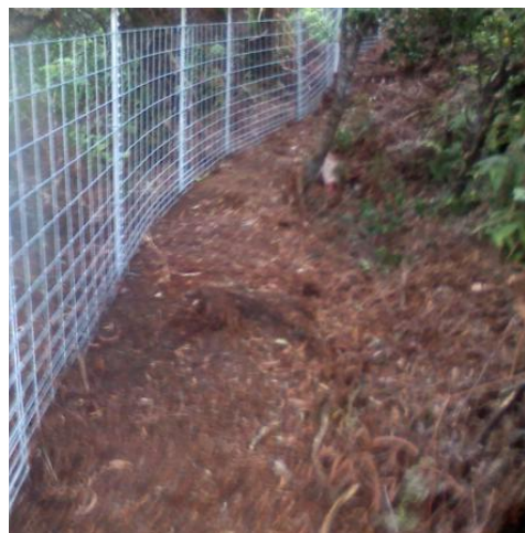
Figure 3. A hog panel fence. The proposed fence would have an additional half panel attached above for an effective height of 7.5 feet.
