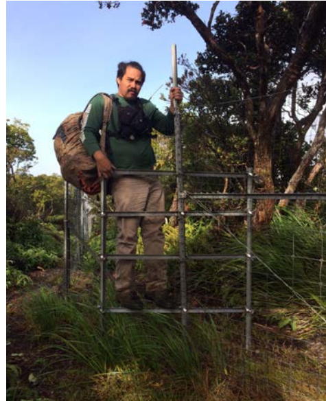
Figure 5. Step-over gate in the EMoWP's Kamakou fence unit allows for continued access to the interior of the fence.
