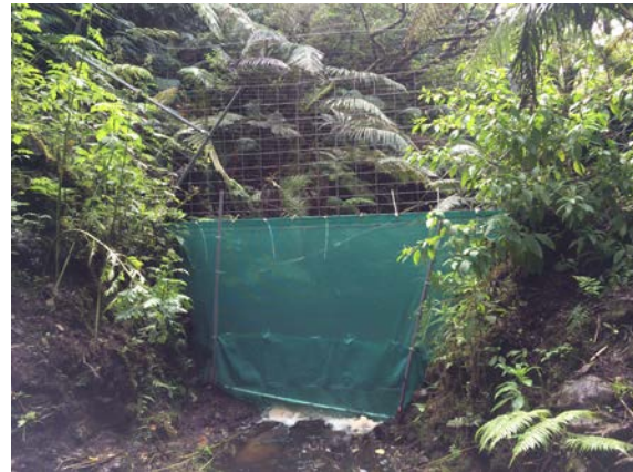
Figure 4. A stream crossing in the EMoWP's Kamakou fence unit. "Break-away" ties run along the sides of the mesh curtain.
