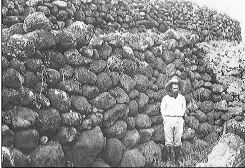
Figure 30. Retaining wall of terrace at heiau in West ‘Ōhi‘a, Site 167. This wall is 3 m (11 ft.) high and the terrace is 45 m (150 ft.) long. Photo by Stokes (1909) as illustrated in Summers (1971).
