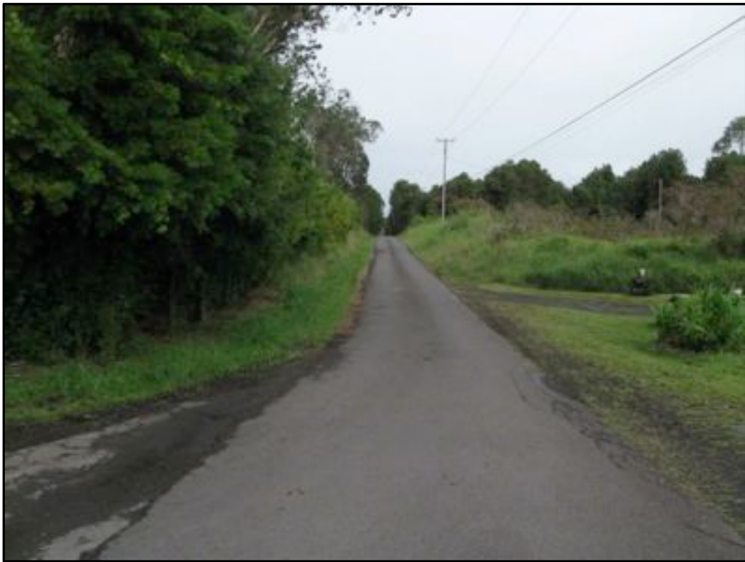
Figure 73. Ihope Road, former path of Site 30088 'Ōla'a Back Road (view to northeast)
