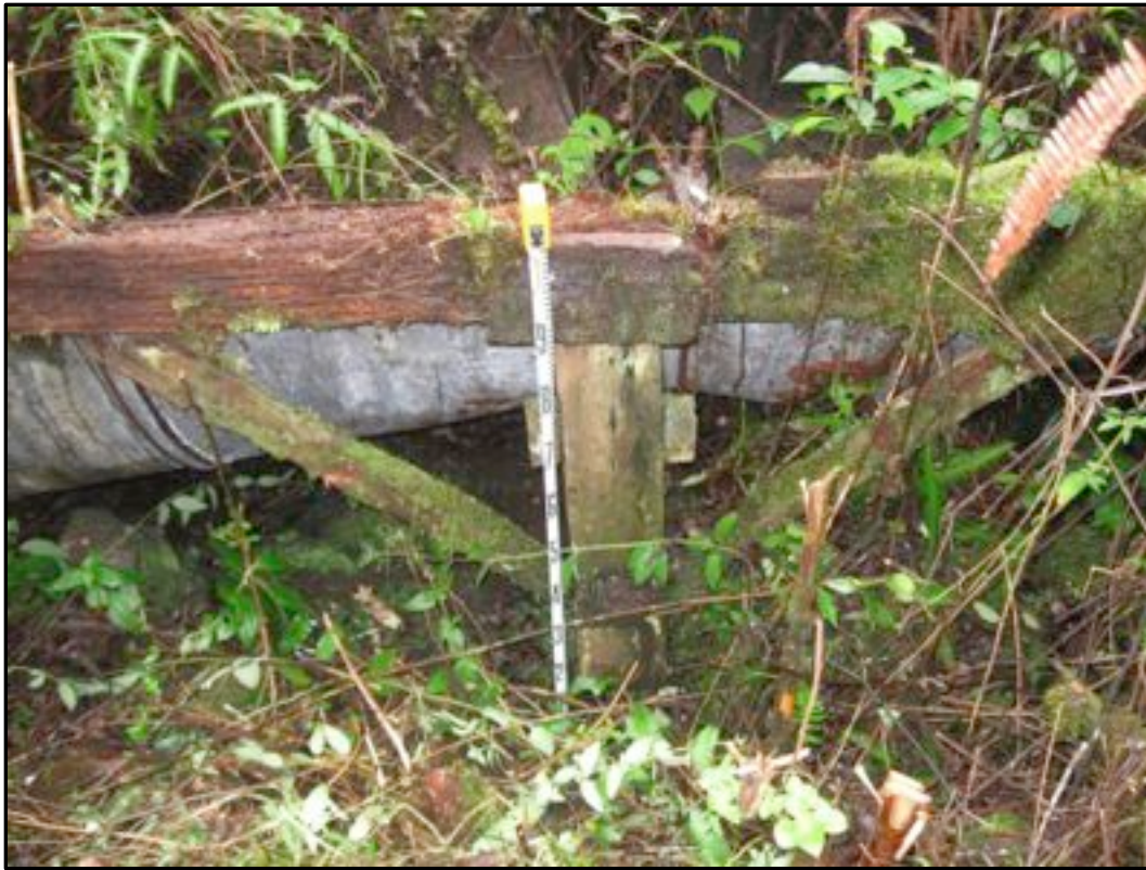
Figure 63. Intact section of Site 20870 Flume (view to northeast)
