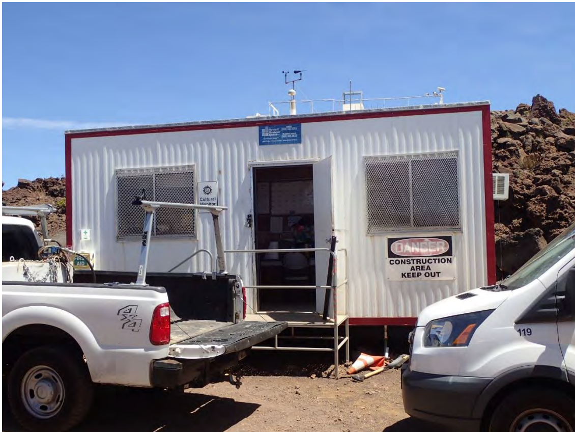
The Construction Site Manager Office trailer was found to be free of non-indigenous invasive arthropods.
