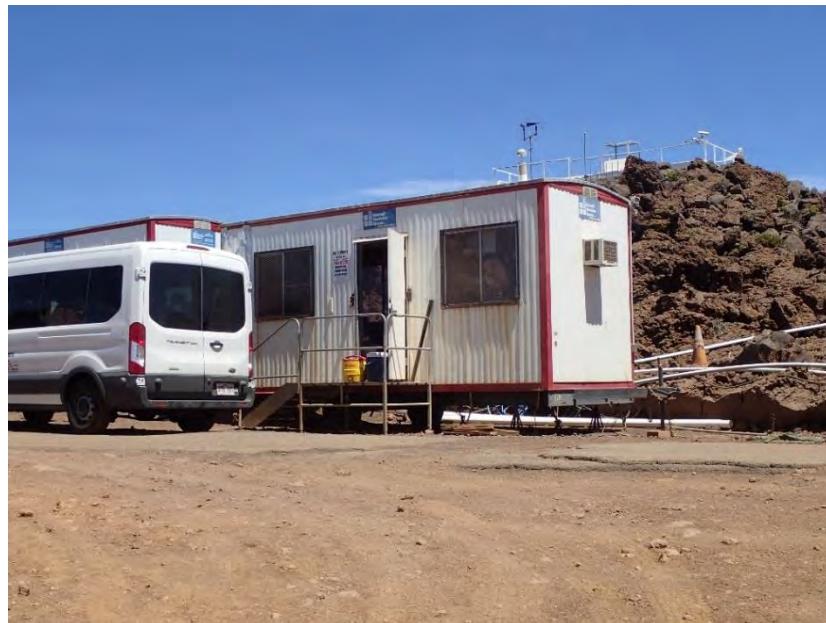
Subcontractor Offices (1 and 2) were clean and no evidence of invasive arthropods were found.
