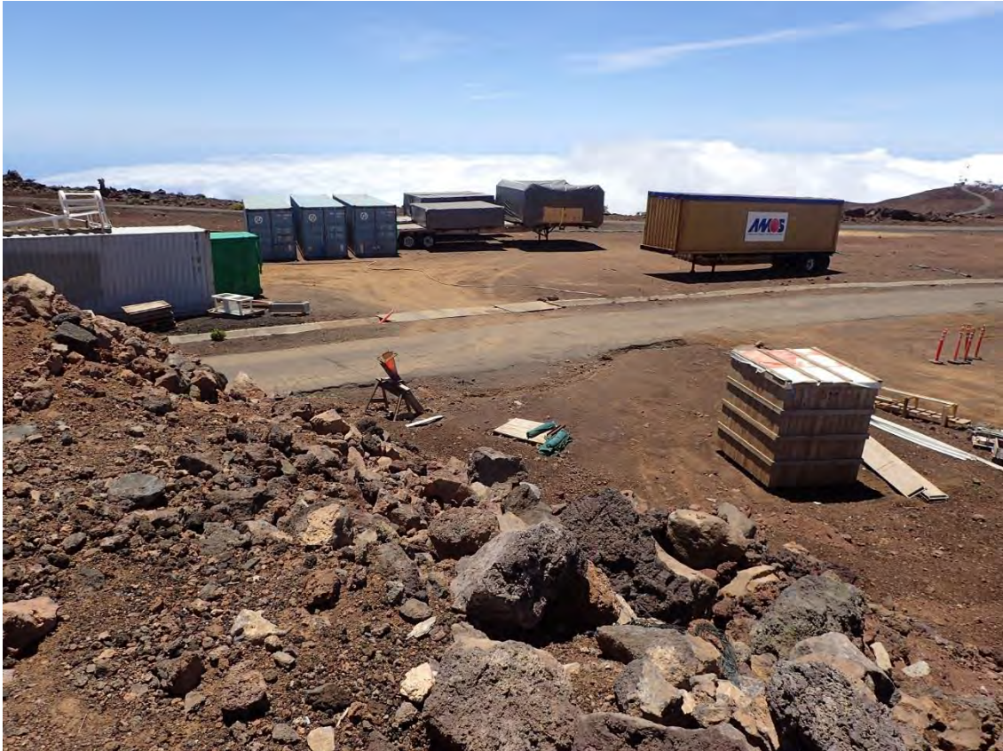
Storage containers at the lower lay-down area were locked and not available for inspection.
