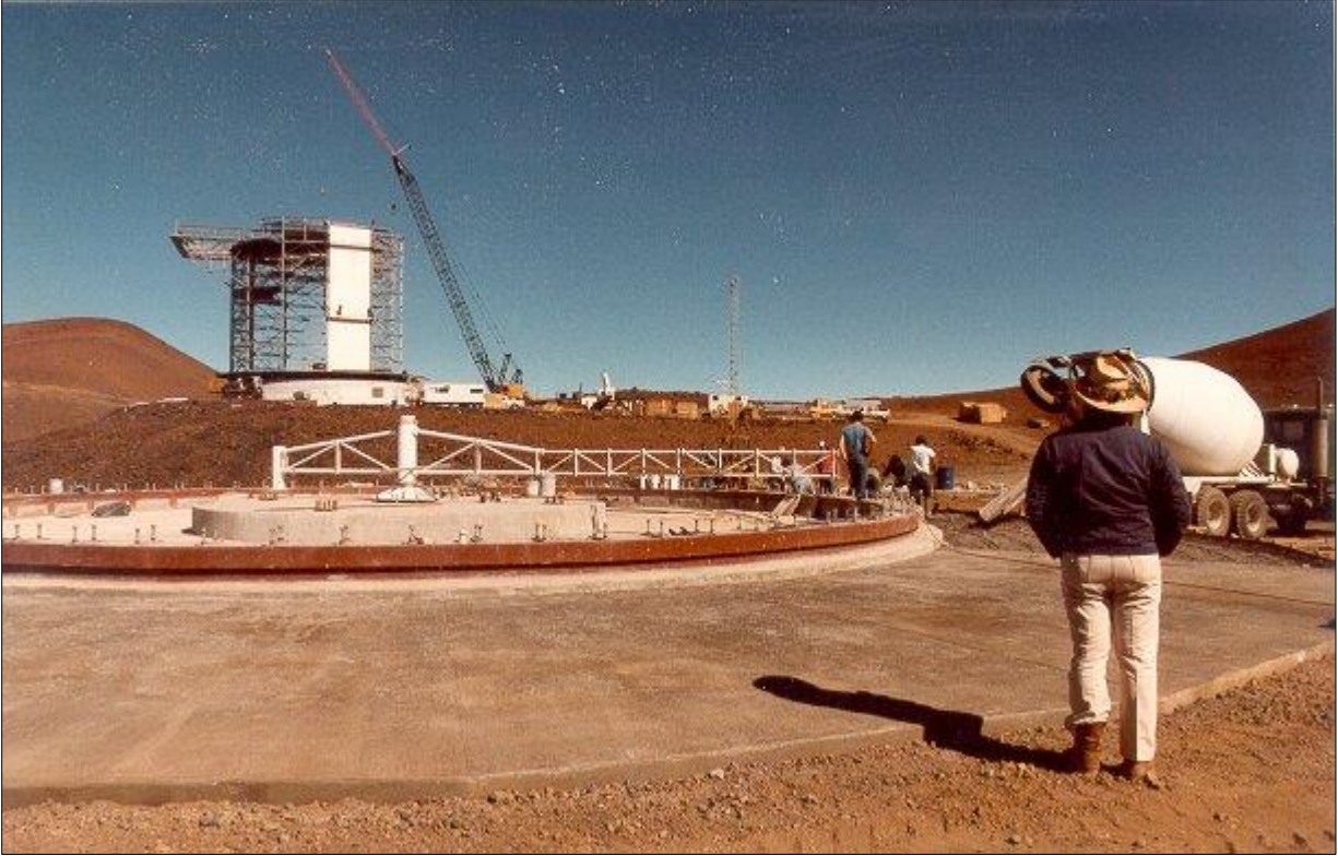
Figure 12. CSO under construction, view to the northwest (Steiger 2009).
