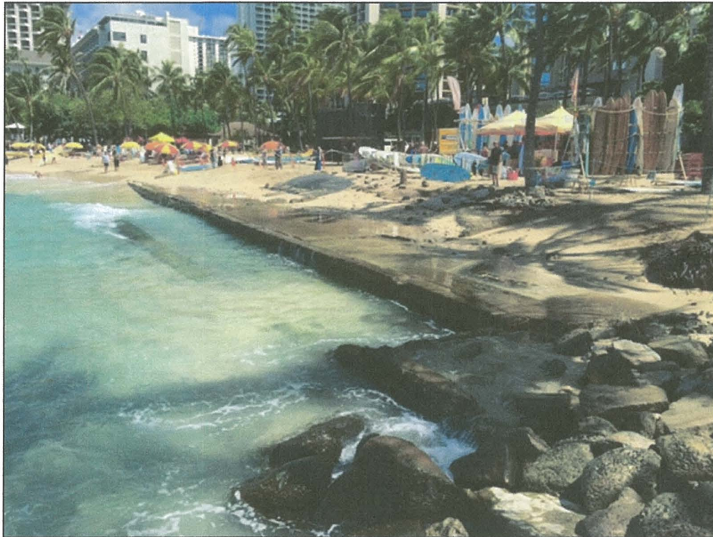
EXHIBIT 6: Exposed Waikiki Tavern concrete foundation (August 21, 2017 photo)
