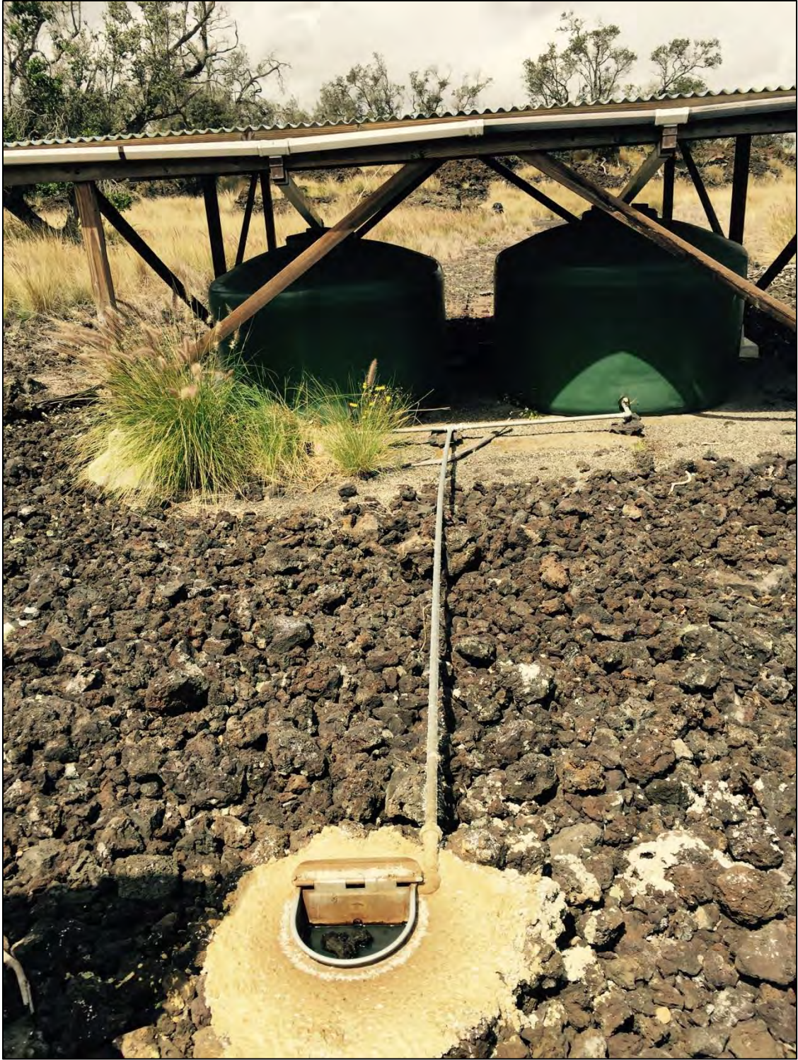
Figure 14.3. Game guzzler located in the PAHGMA. Float valve and trough in the foreground, connected to the catchment system pictured in the background.
