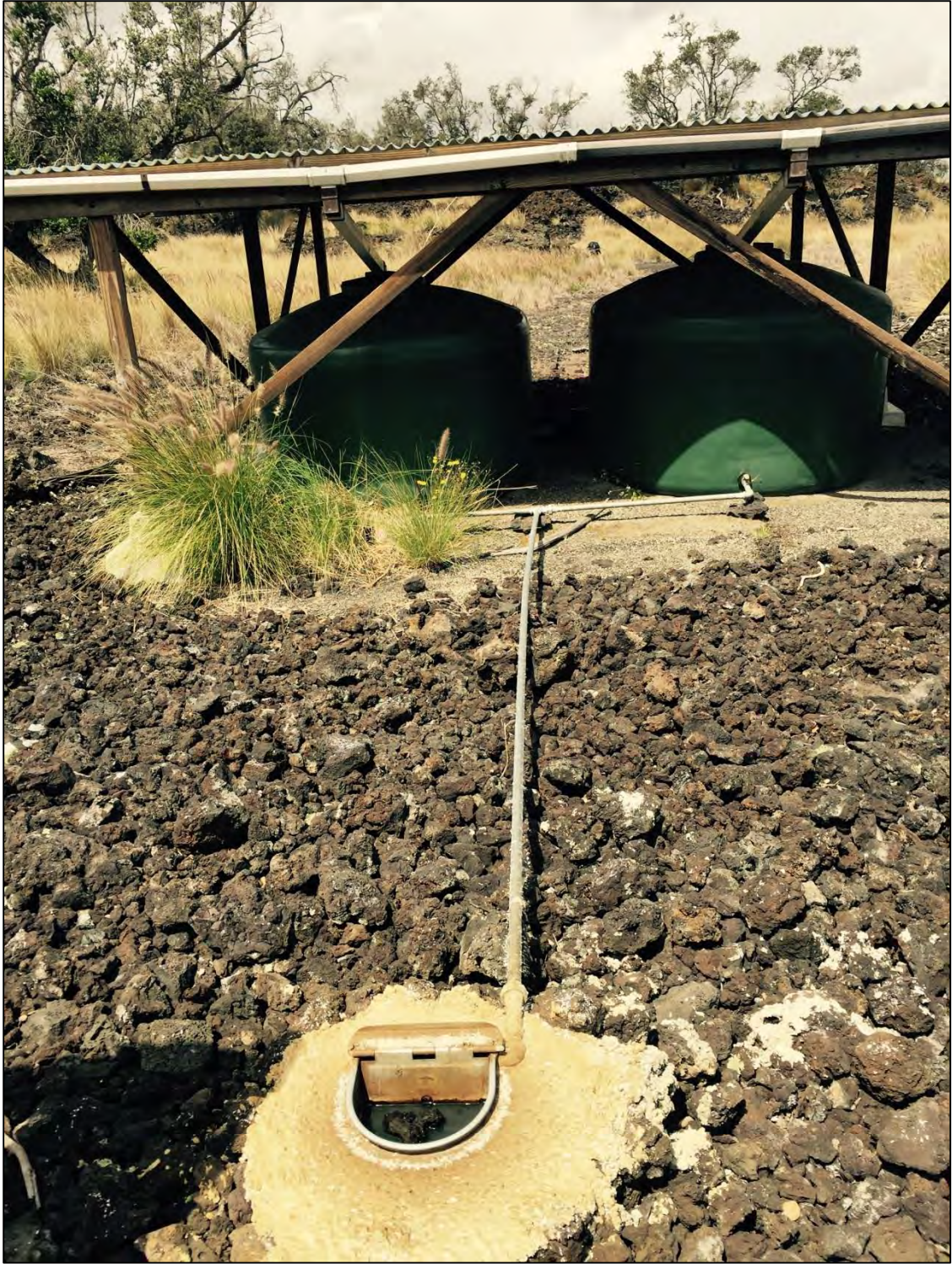
Figure 1.4 Game guzzler located in the PAHGMA. Float valve and trough in the foreground, connected to the catchment system pictured in the background.
