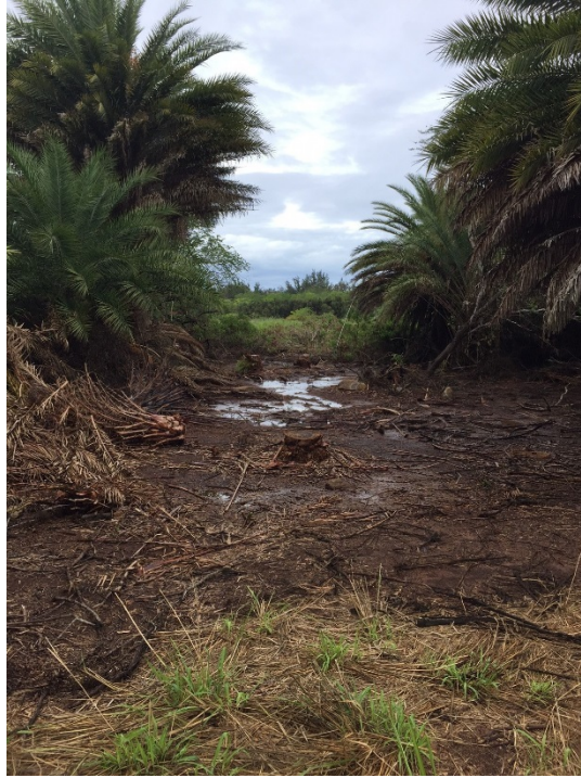
Figure 5: Bat Lane Constructed at ‘Uko‘a Wetland.
