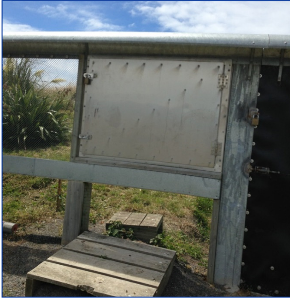
Figure 10.3. Example of pedestrian gate design that does not extend to ground level (Young and VanderWerf 2014)
