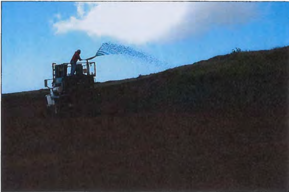
Figure 1. Mechanized hydroseeding along a bare road cut during immediate site revegetation and soil stabilization efforts following construction at KWP.
