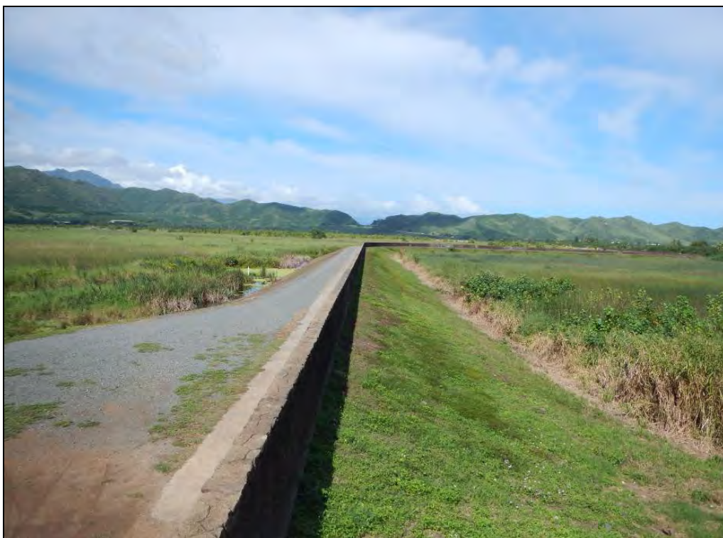
Figure 84. Kawainui Marsh levee and trail, view to north
