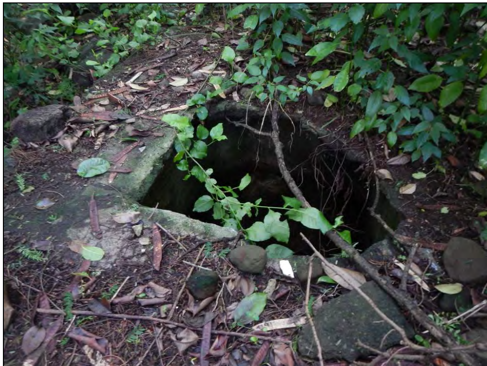
Figure 90. Concrete well structure, view to northeast
