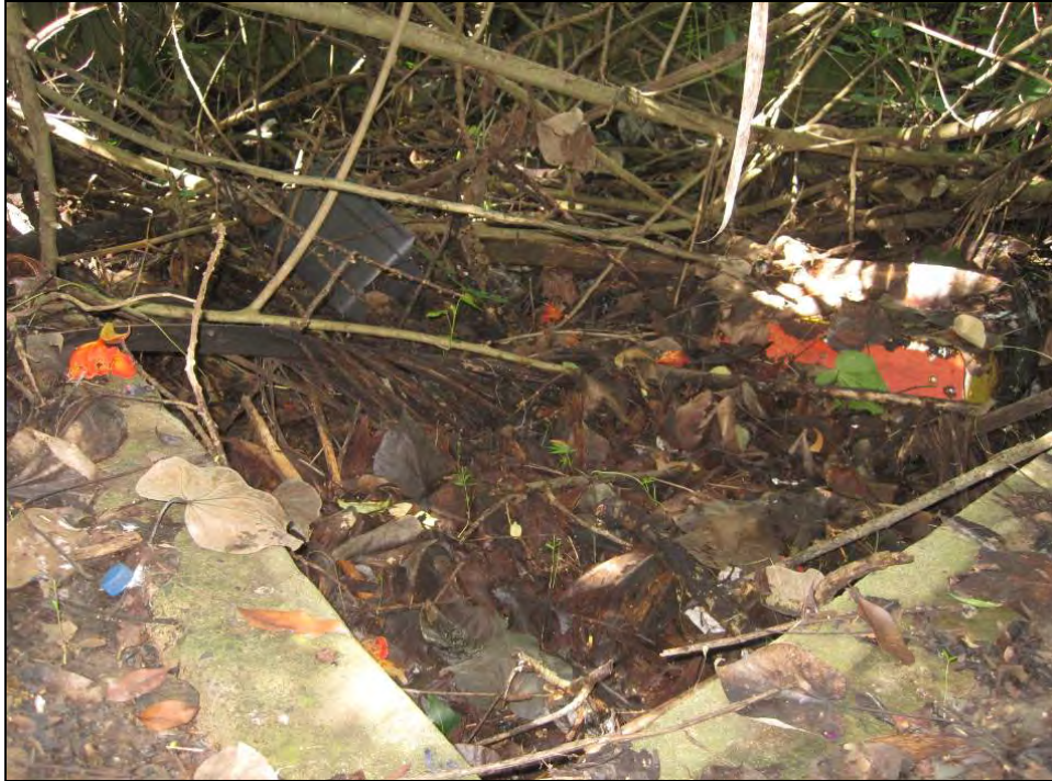
Figure 87. SIHP # 50-80-15-4042, rectangular northern portion of the Waimanalo Irrigation System pump house, view to southeast
