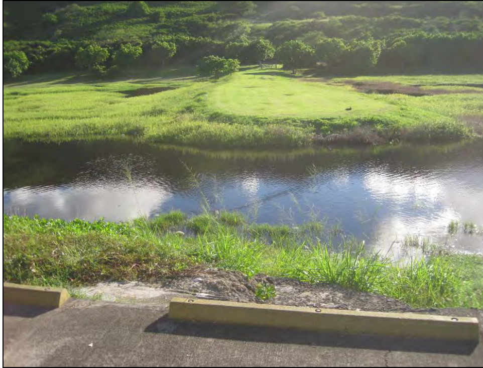
Figure 65. Abandoned road corridor that extends north/south through Hāmākua Marsh, view to south
