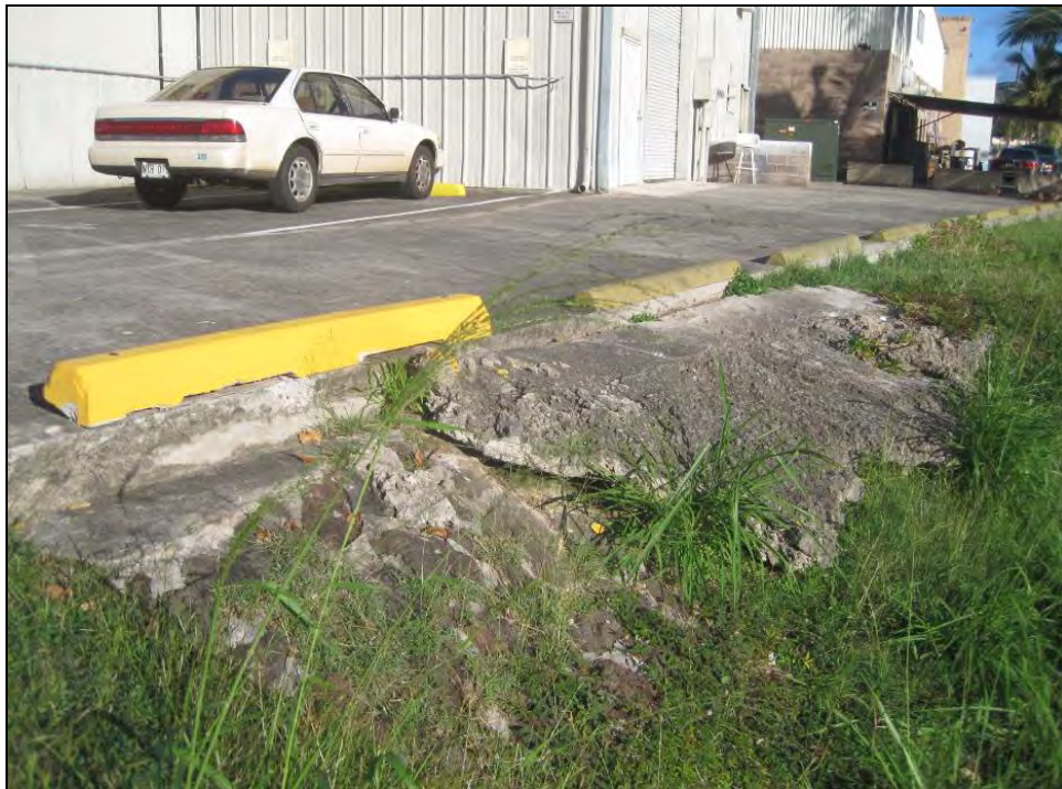
Figure 66. Asphalt and rock and mortar remnants that may have supported a bridge or road extension leading from Hāmākua Drive to the abandoned corridor, view to southeast
