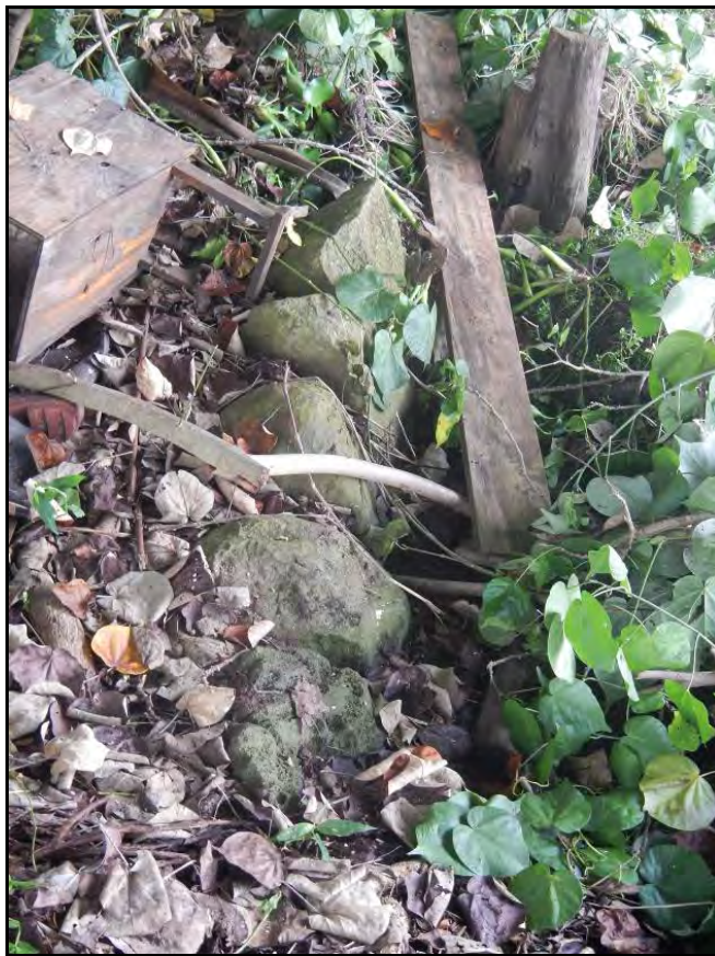
Figure 132. Basalt wall section at Nā Pōhaku o Hauwahine, view to southeast
