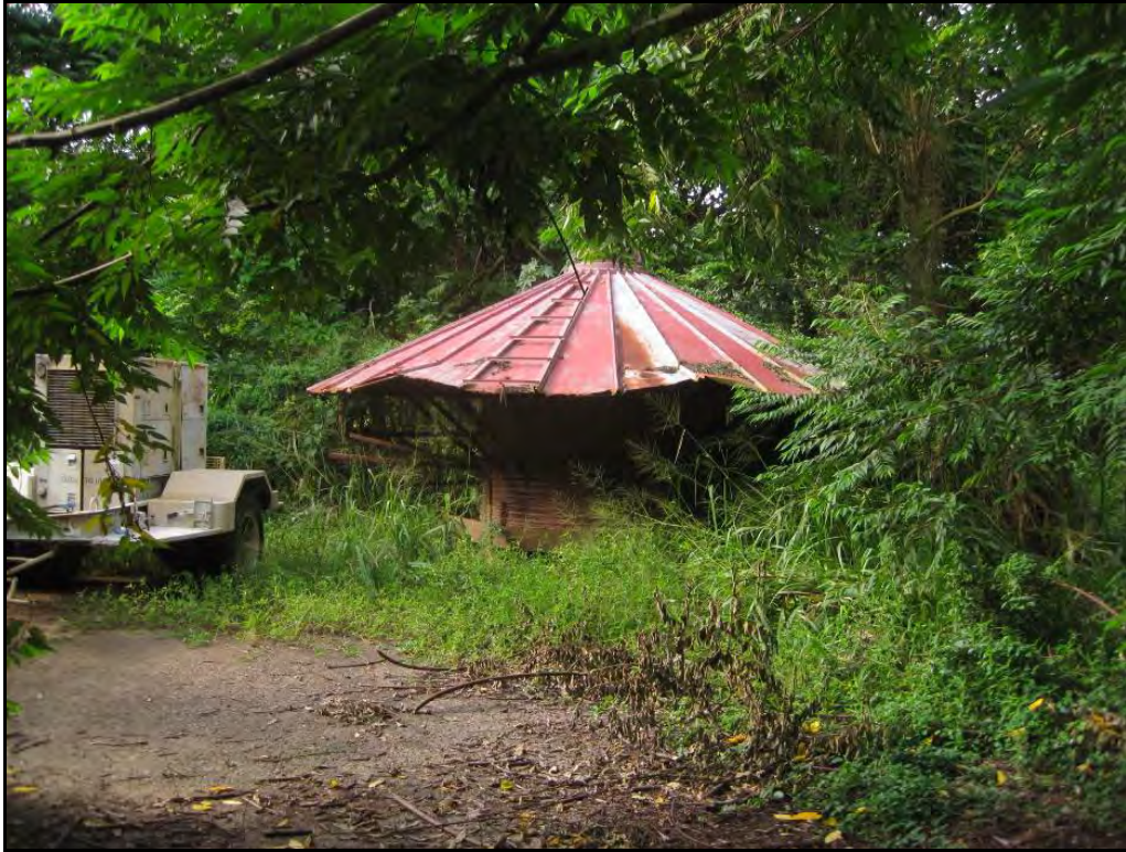
Figure 111. Former Knott's Ranch cattle feeding station, view to east
