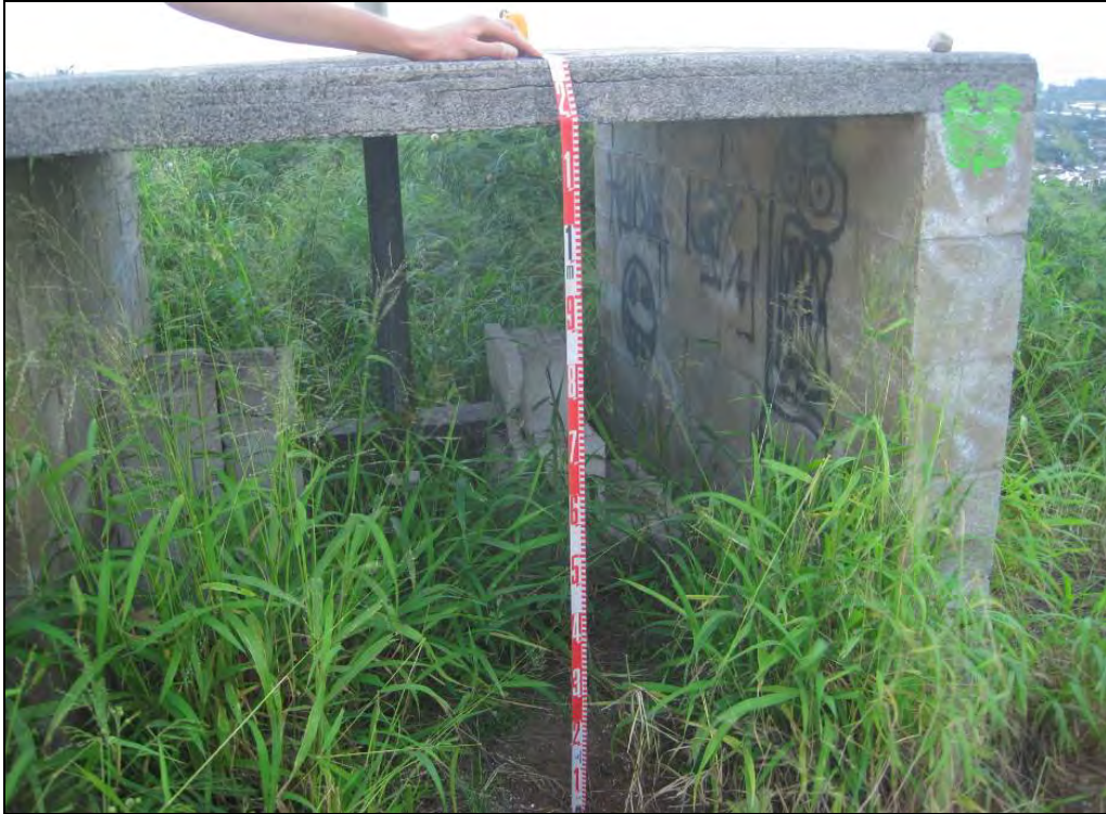
Figure 75. Triangulation station, view to east
