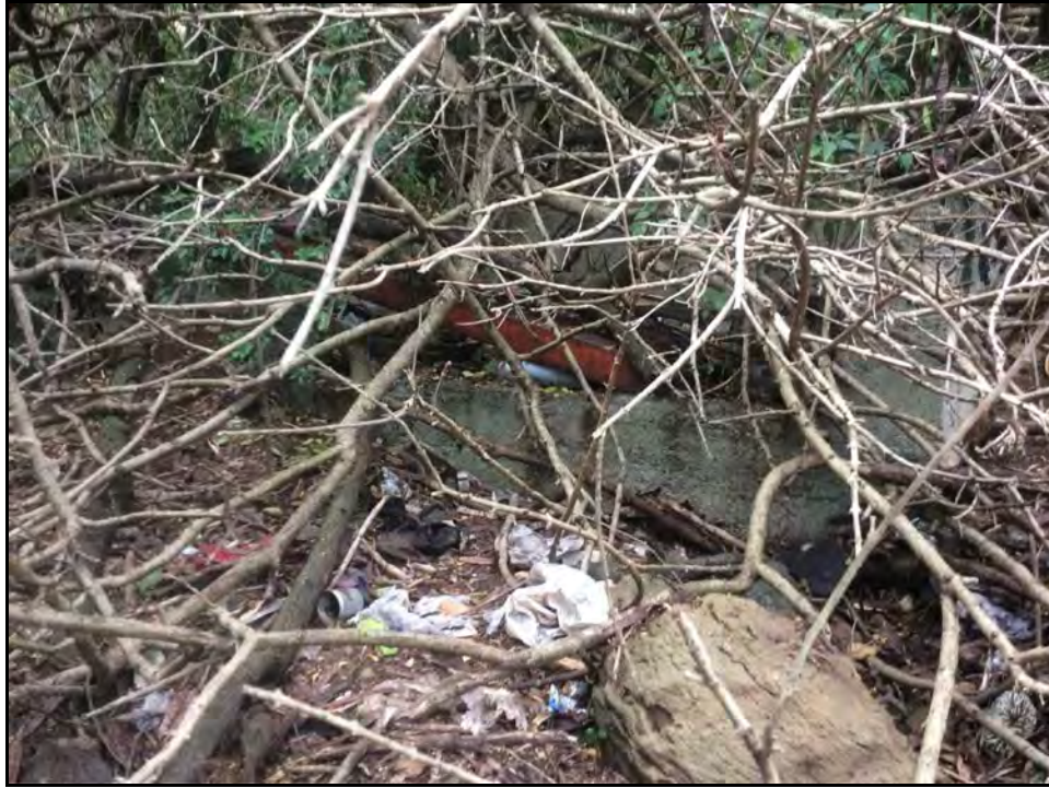
Figure 59. Photograph of CSH 5, concrete structure of unknown function, view to southeast
