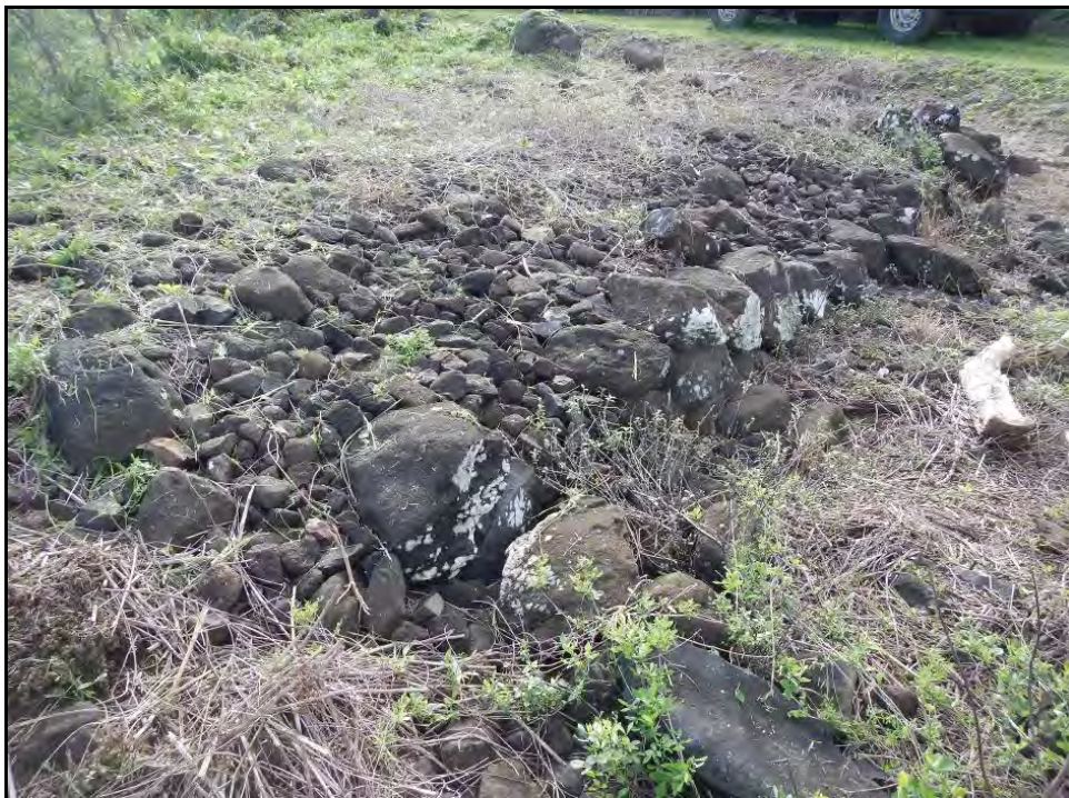
Figure 60. Section of a faced wall, appears to be in the same location as SIHP # -4428, habitation complex, view to southeast
