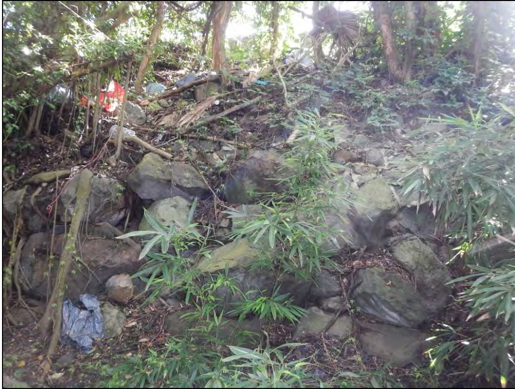
Figure 89. Basalt boulder retaining wall downslope of Kailua Road, view to east
