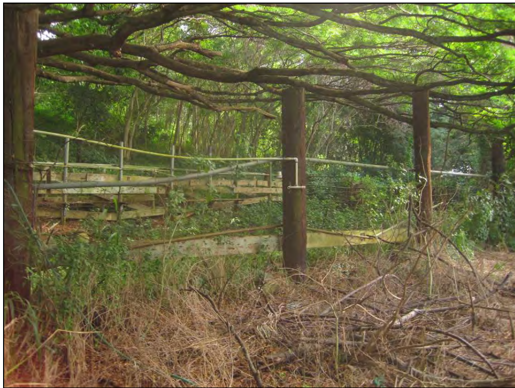
Figure 110. Former Knott's Ranch corrals located east of the DOFAW campus, view to west
