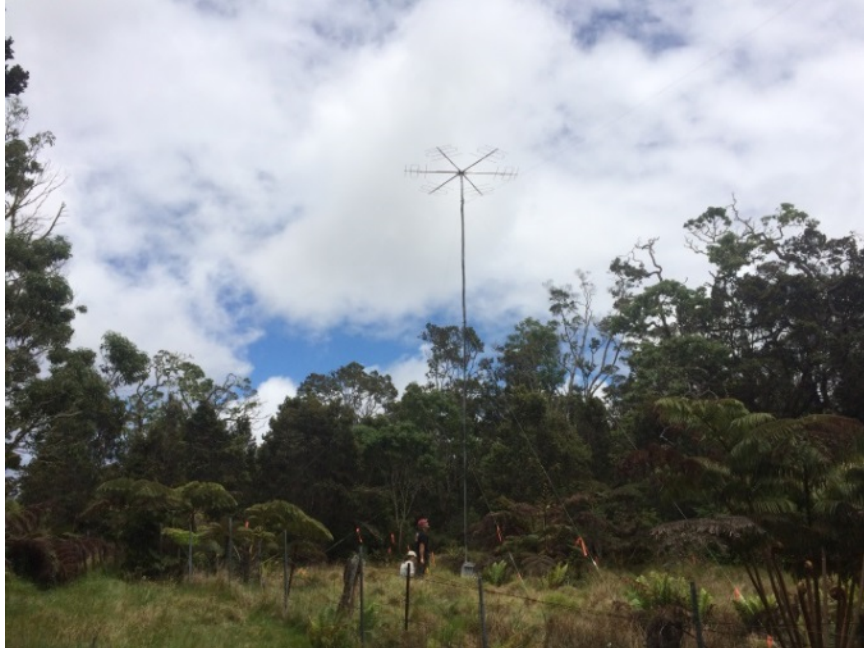
Figure 2 Forty foot telemetry mast at Hakalau Forest NWR.
