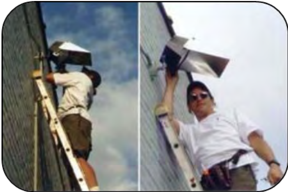
Figure 2: Installation of an appropriately sized floodlight shield. Source: www.darksky.org .
