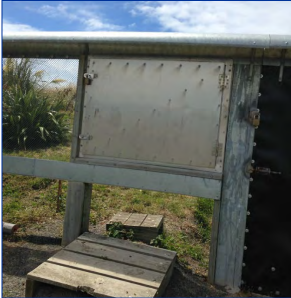
Figure 10.3. Example of pedestrian gate design that does not extend to ground level (Young and VanderWerf 2014)
