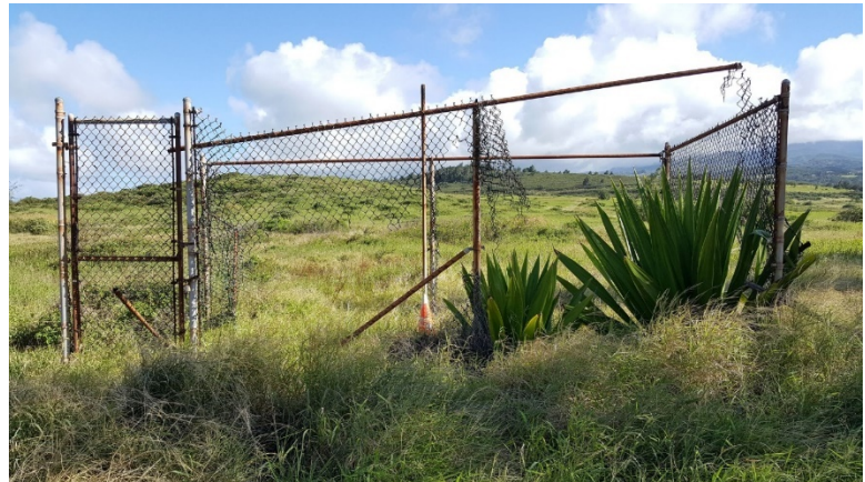
Remnant irrigation pump site adjacent to the Līpoa Point foot trail.
