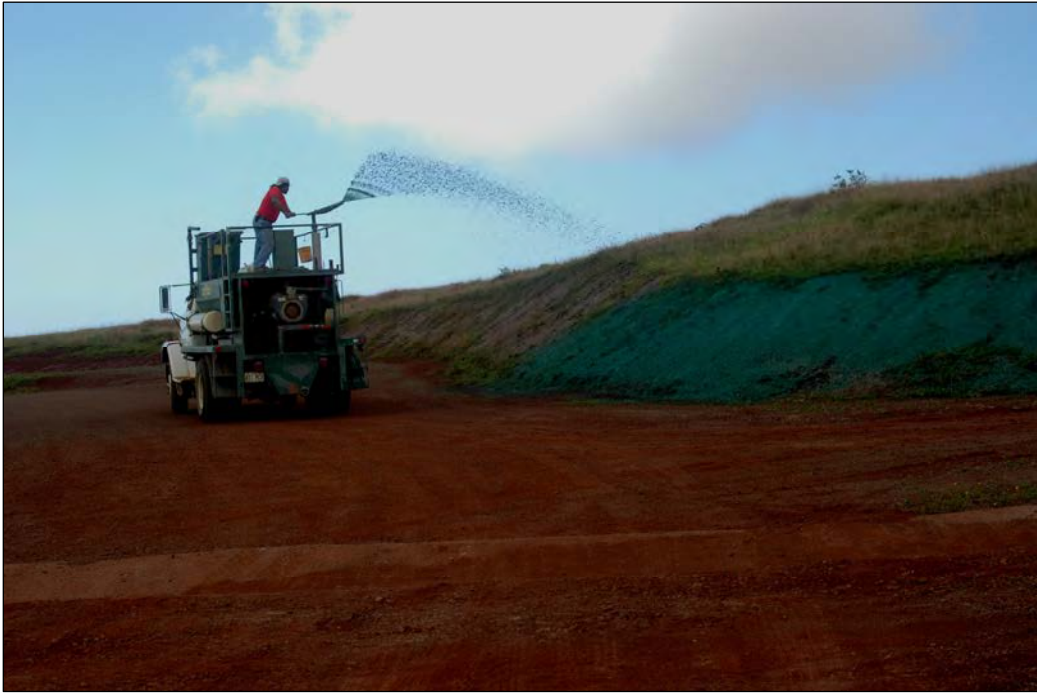
Figure 1. Mechanized hydroseeding along a bare road cut during immediate site revegetation and soil stabilization efforts following construction at KWP.
