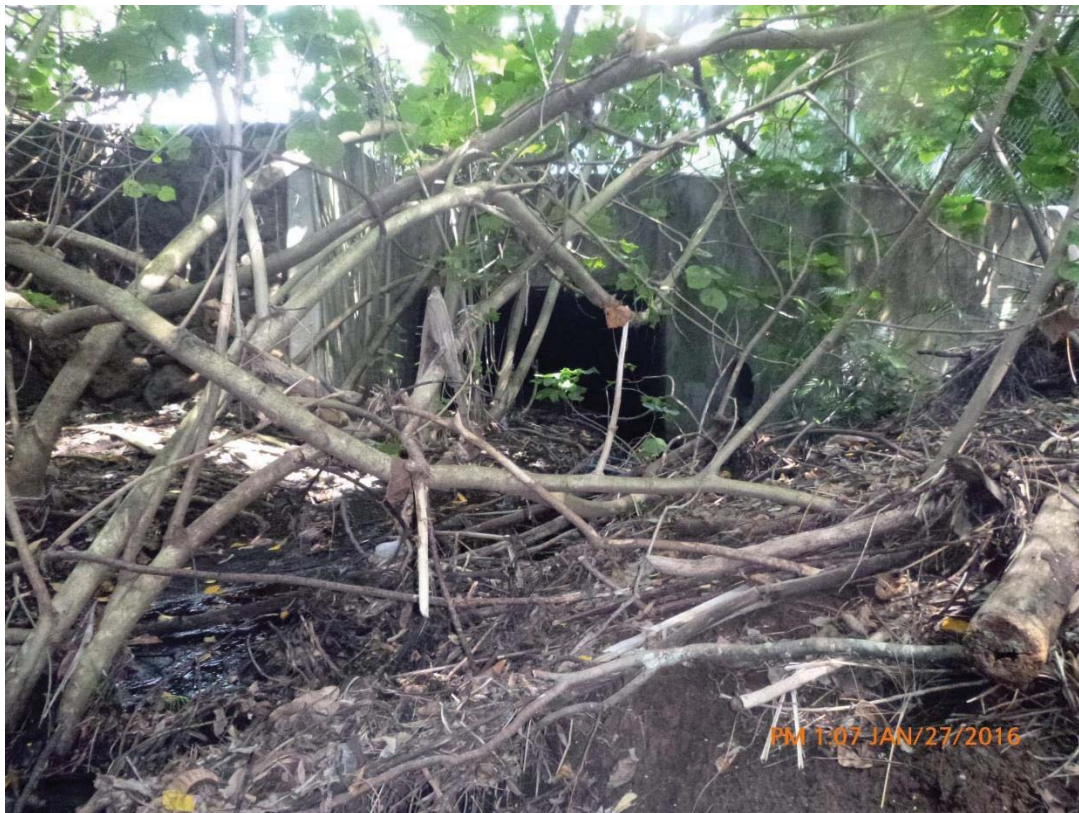
Figure 5. A box culvert discharges groundwater and storm water into Mānoa Stream in the Project area.
