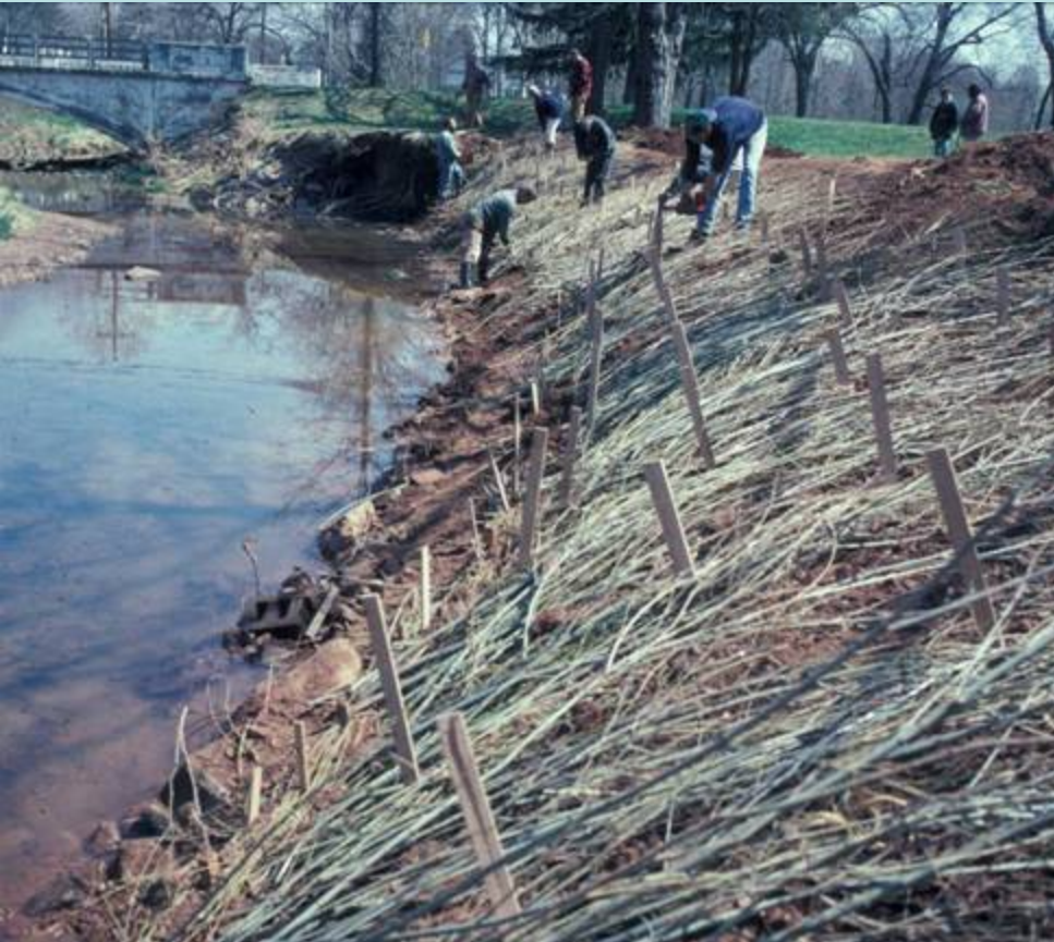
Installation of brushmattress
