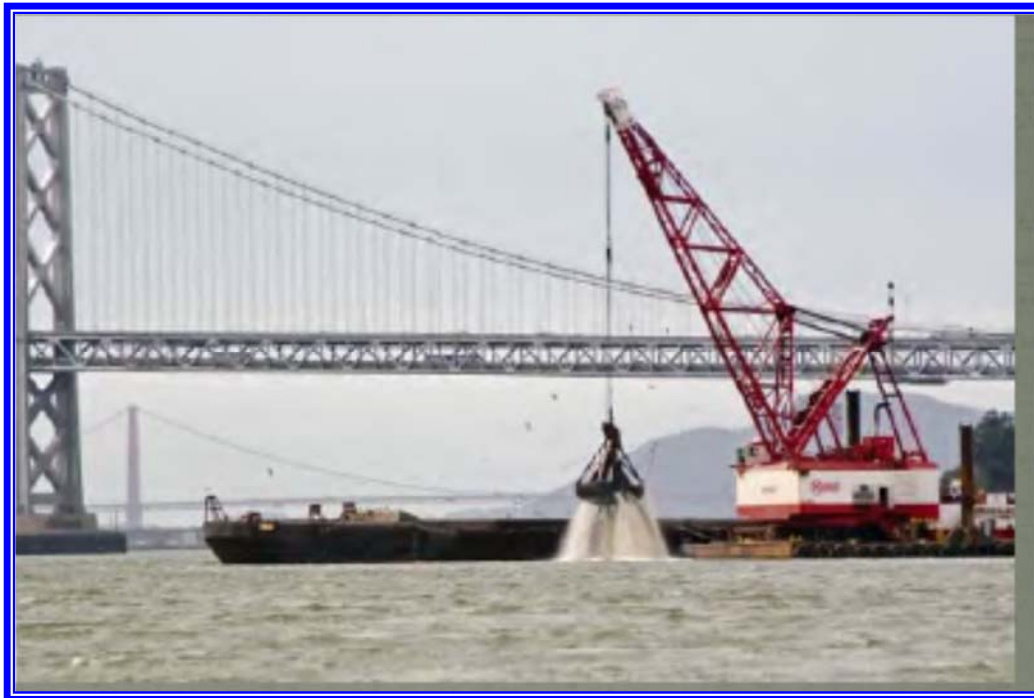
Figure 5-4. Clamshell Dredging Operations
