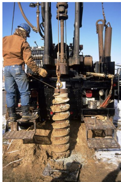
Drilling to monitor for VOCs near a Wisconsin landfill. Photo: DNR
