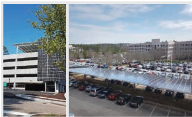
Solar panel installation at Lenovo Morrisville, North Carolina facility - February 2020.
