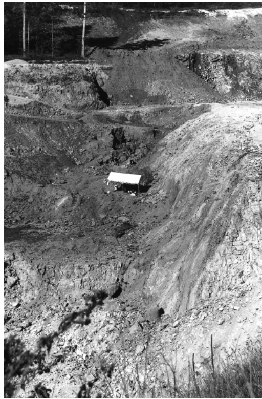
Fig.2 - Bollschweil. Overview of the excavation looking toward the northwest, October 1997.
