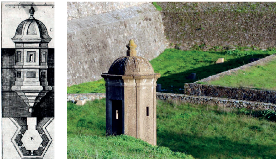
Gatehouse design. Miguel Sánchez Taramas, Cit., Sheet XIV. Gatehouse above the ditch and facing a ravelin and covered way. Photo by N. Gutiérrez Montoya.
