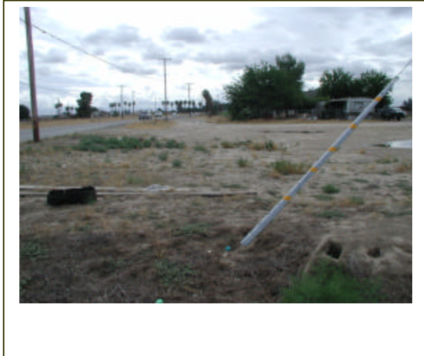
Low pressure gas line location at the southeast corner of Highway 119 and Ashe Road. Facing east.
