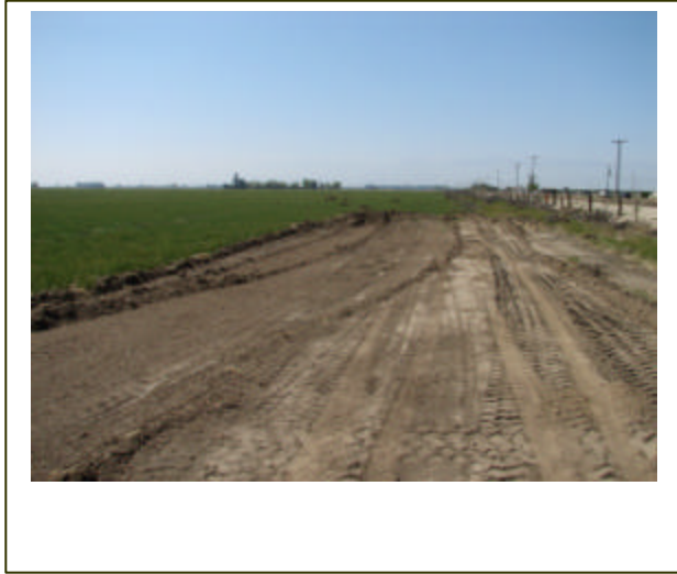
Northwest corner of project site, facing south
