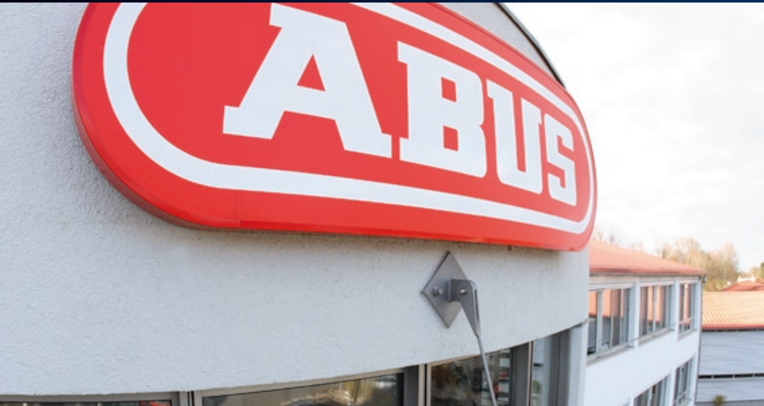
Company headquarters ABUS Security-Center in Mühlhausen near Augsburg (Germany)
