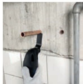
Flush cutting of a protruding copper pipe.
