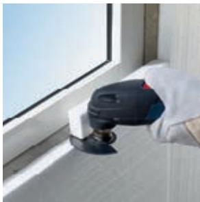
Flush cutting to length of protruding insulation material, e.g. polystyrene.
