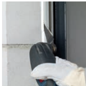
Cutting soft expansion joints.
