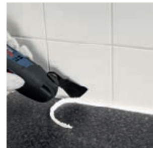
Removing old silicone joints.
