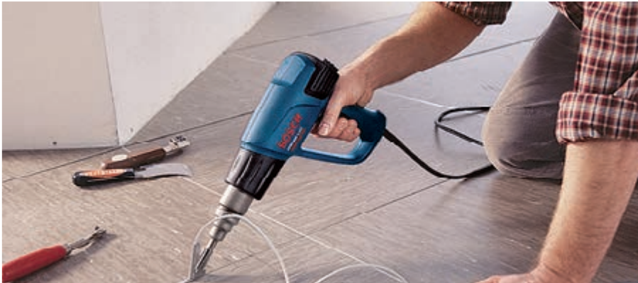
Joints can be welded with the welding shoe
