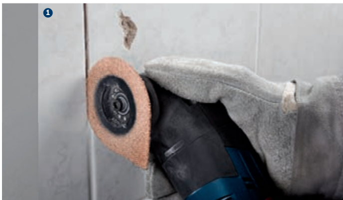
1 Routing joints on wall and floor tiles
