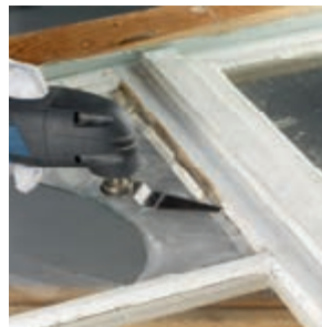
Cutting window putty (sealing compound).
