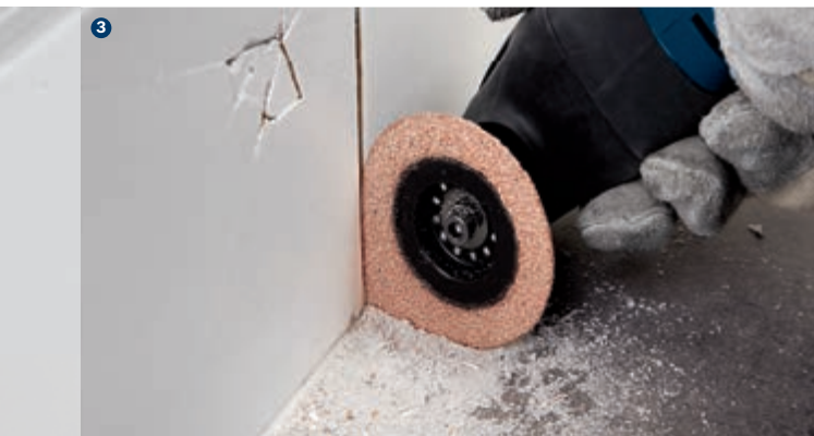
Routing joints right into 90 degree corners
