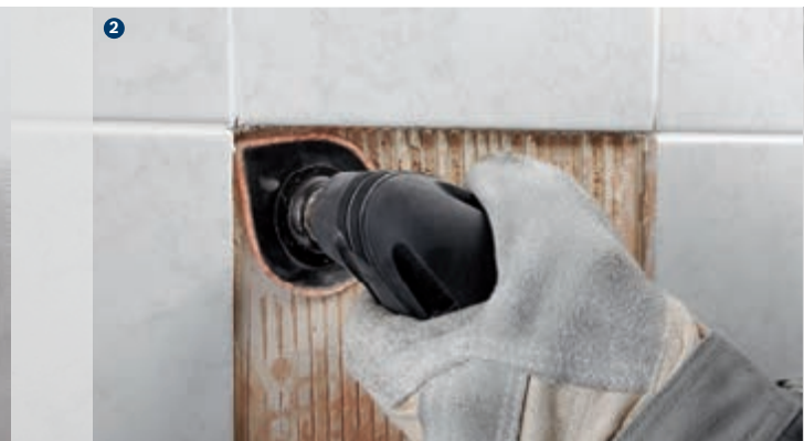
2 Removing mortar or tile adhesive – even right into corners
