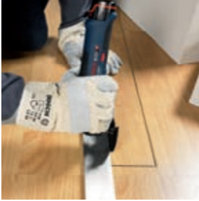
Precisely cutting out laminate/parquet, e.g. for installing a partition wall.
