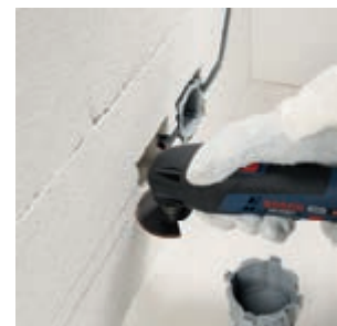
Routing grooves in porous concrete, for laying concealed cables and pipes.
