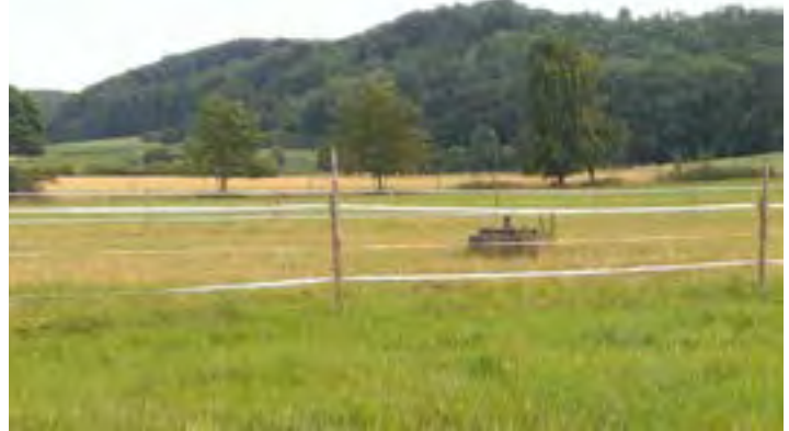
Figure 3-26. Typical facility for drinking water extraction from springs; in maps one often finds “Wbh.” (Wasserbehälter) as its topographical signature.
