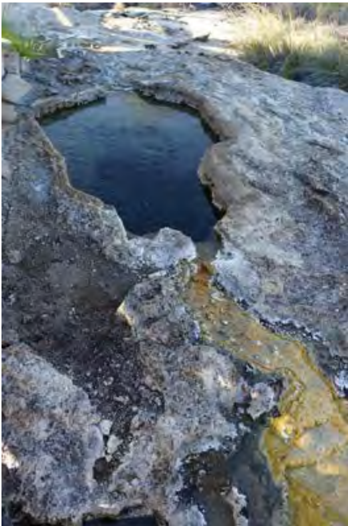
Figure 8-99. Physical damage in the form of grooving of the lip of the spring vent to guide the direction of water flow around the travertine mound at Talaroo Hot Springs (photo by Peter Negus).
