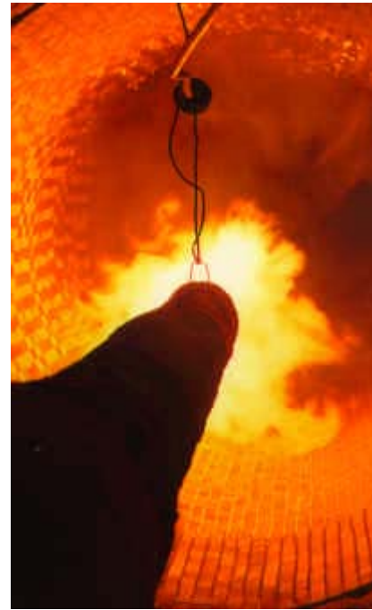
Inside a cement kiln, where temperatures reach more than 1400°C (2550°F).
