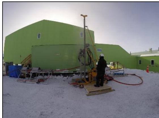
Figure 20: Drilling during Hillary Field Centre Site investigations.
