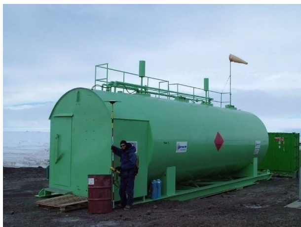
Figure 8: Bulk JP8 fuel tank, Scott Base
