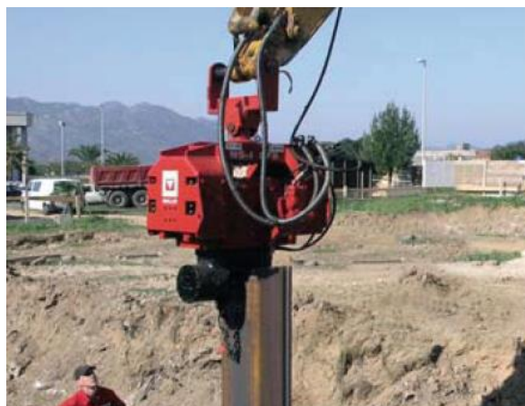
Figure 27: Vibro-hammer used to install piles
