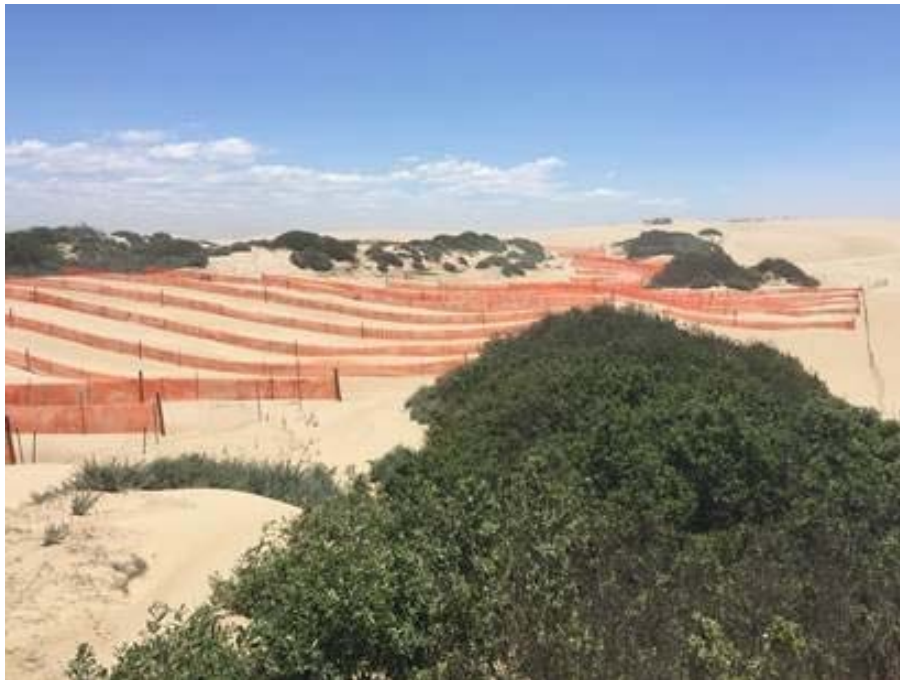
Photograph 12: Dust control program wind fencing at Tabletop
