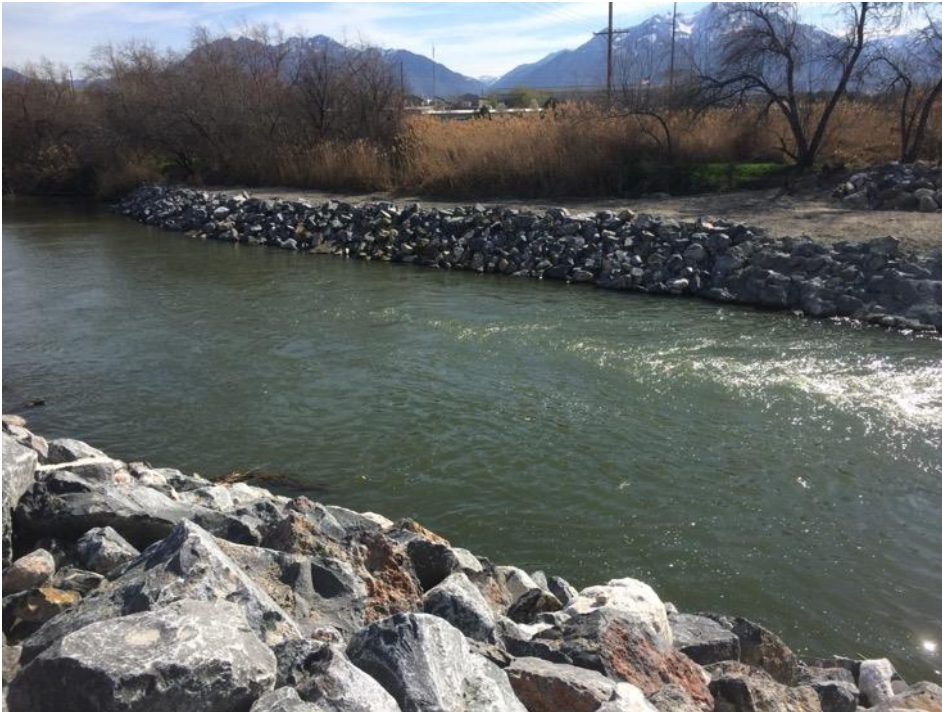
Appendix 8. Jordan River bank stabilization rip rap.
