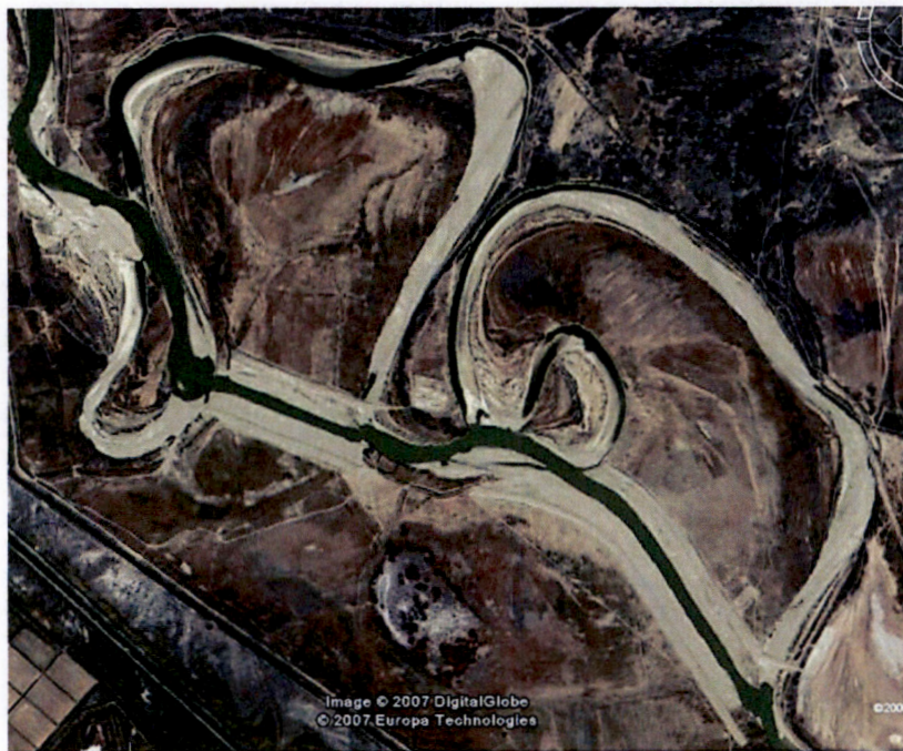
Fig. 1-3: Google Earth image of completed riverbed straightening under SYNAS-I (Contract 006a)
