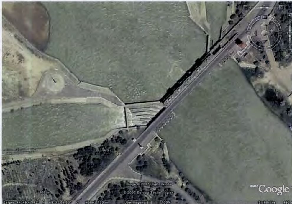
Fig. 5-1: Overview of the location of the subproject at Google Earth satellite image.
