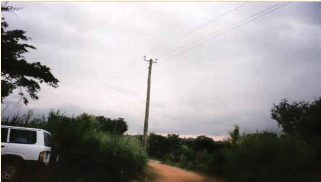
Note | A ground conductor is strung under the two insulated phase conductors, for multiple earthing. Photographed by Prof. Francesco Iliceto.
