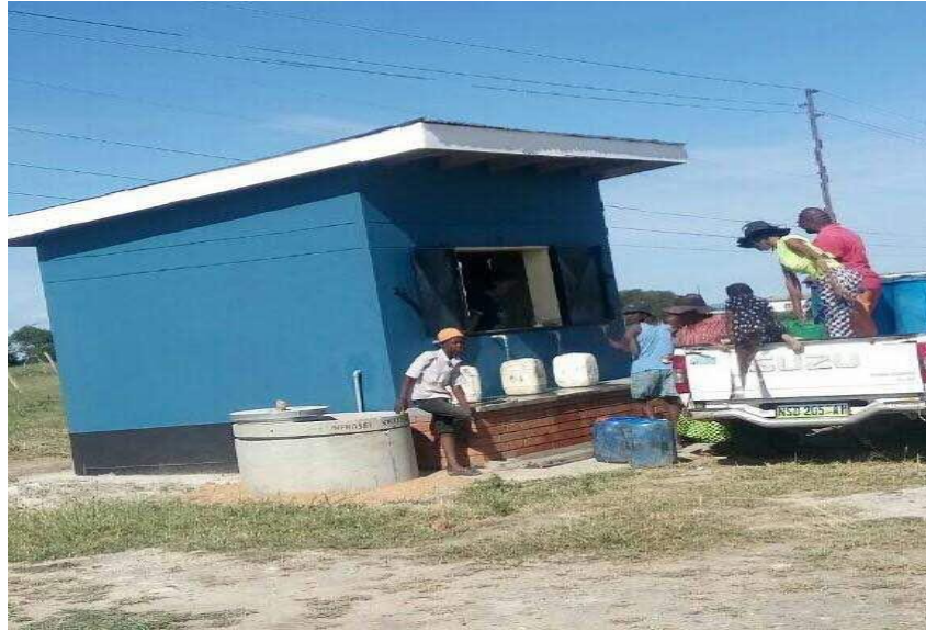
Photoplate 5: Water Kiosk in Operation
