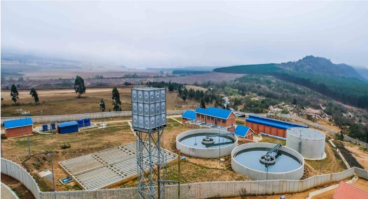
Photoplate 2: Existing Masibini Water Treatment Plant
