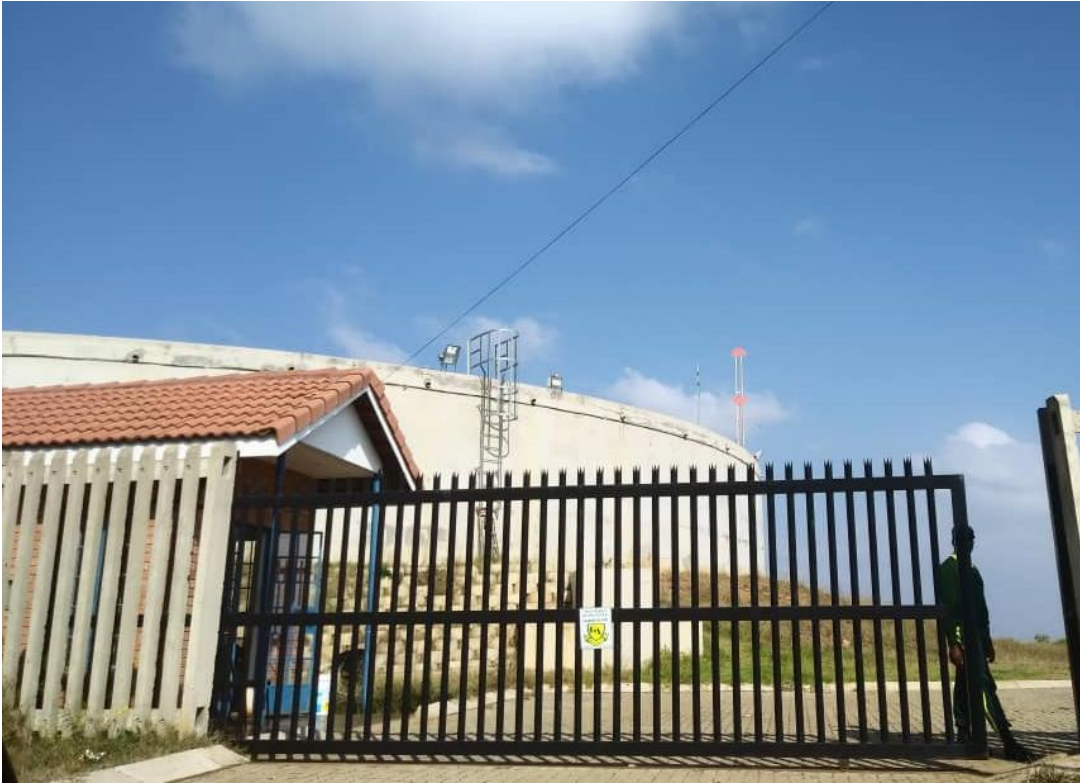
Photoplate 4: Existing Masibini Reservoir
