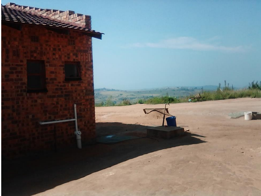
Photo plate 26: Long awaiting plumbing
