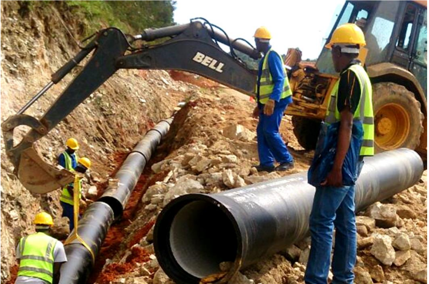
Photoplate 3: Typical Pipeline Installation
