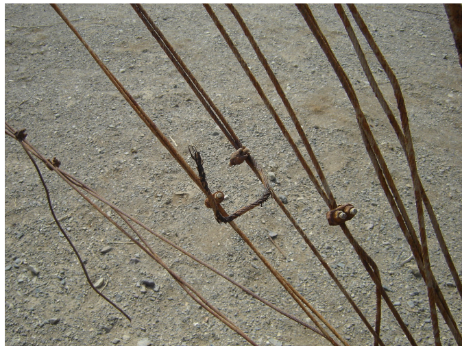
Figure 5-7: Tilted metrological mast near the project site Figure 5-8: Rusted steel wires of the metrological mast
