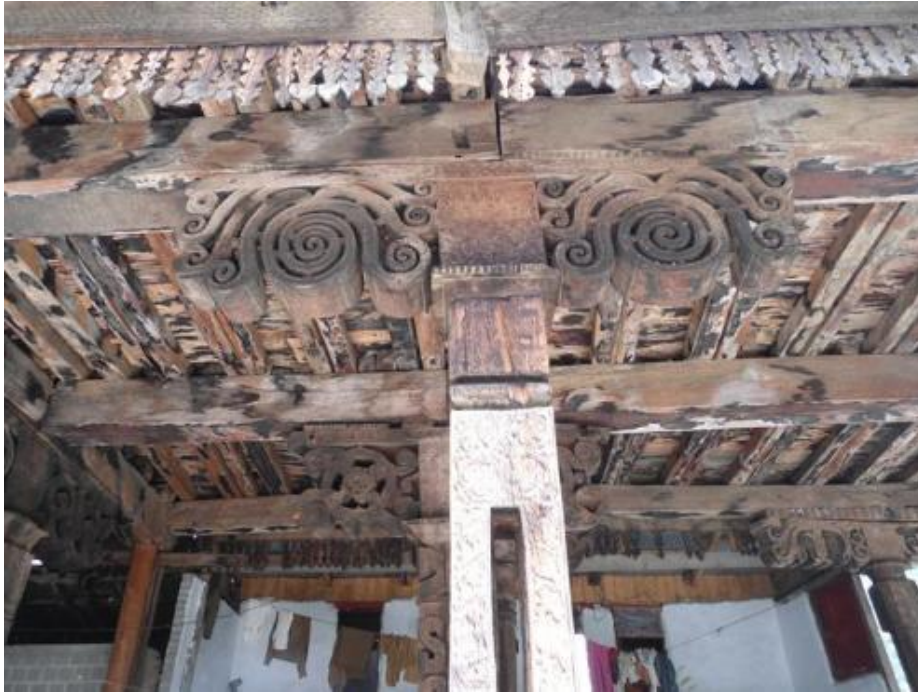
Figure 5.8: Seo Mosque showing Wooden Pillar and Brackets
