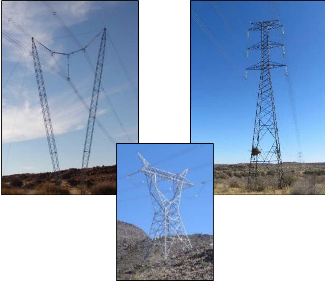
Figure 2. The structure of the pylons for the planned 400 kV power line, showing the V-type guyed (cross rope) suspension tower (used for 90% of the line) (left), and the self-supporting strain structure (inset); and the self-supporting pylon of the existing 220 kV power line (right); the structure for the 220 kV strain towers is similar.
