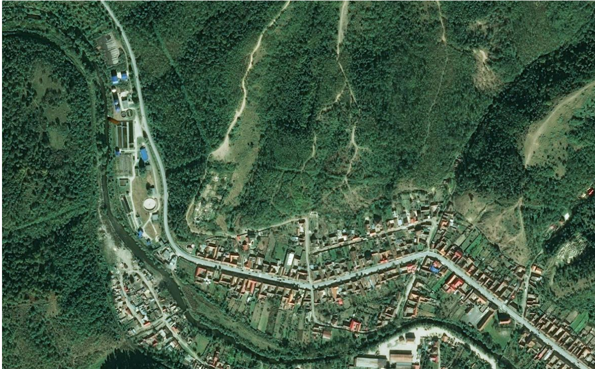
Figure 68 – Reșița Wastewater Treatment Plant Source: Google Maps
